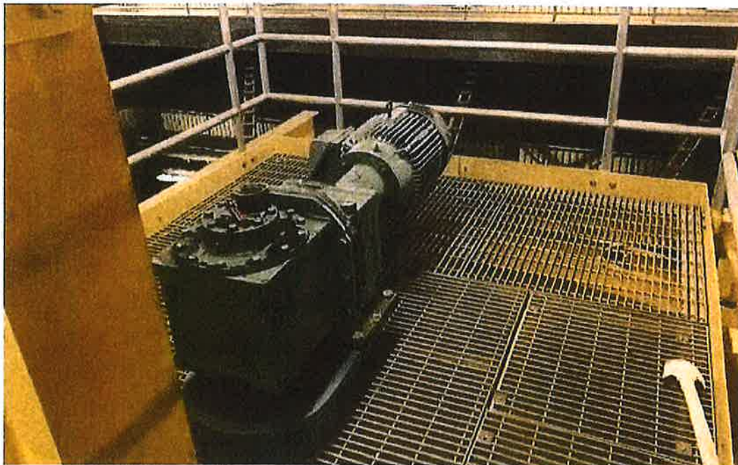
Picture of heavy-duty drive unit for a softening basin mixer in the 1997 Lime Softening Water Treatment Plant (LSWTP). These drives are 25-year old and original to the LSWTP. The drives will be replaced with new ones in project WA2152.
