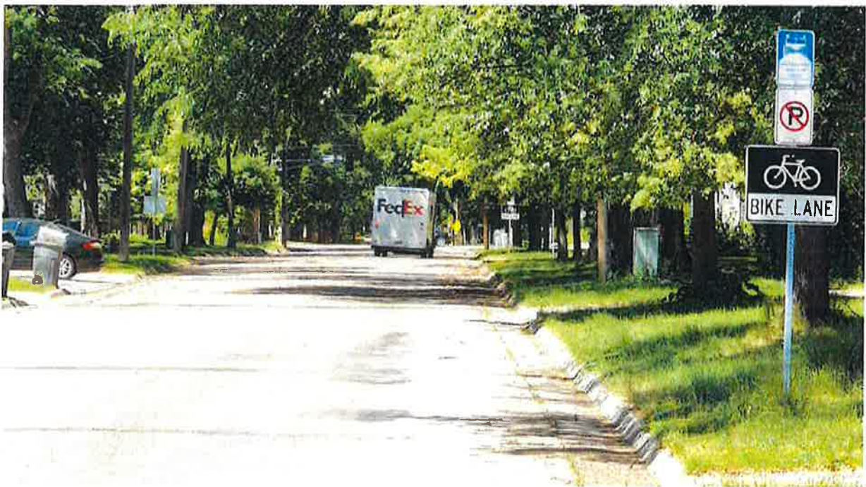
The painted bike lane along 7th Ave in Moorhead is no longer visible; periodic re-application of paint is required to maintain this facility.
