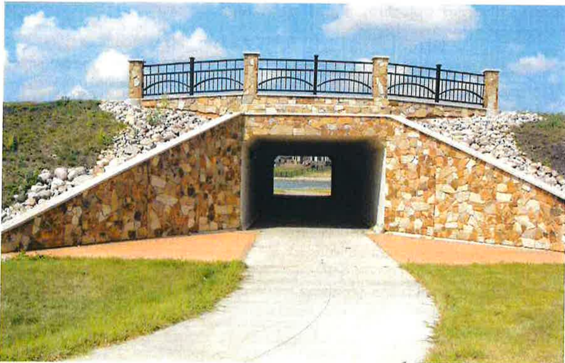
An existing trail underpass in West Fargo
