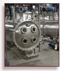
Water from the Red River is hard (high mineral content) and the water treatment process centers around softening the water (removing minerals). This process reduces hardness from an average of 17 grains per gallon to a target value of 7 grains per gallon. The residual hardness in the finished water prevents the water from becoming too corrosive.
