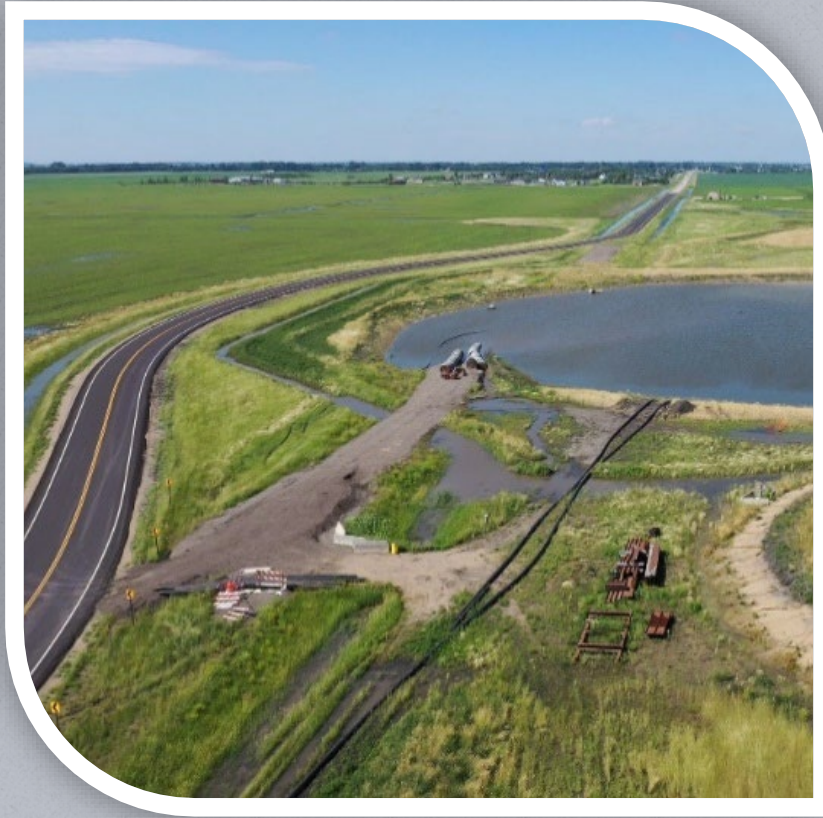
FARGO-MOORHEAD AREA FLOOD DIVERSION
