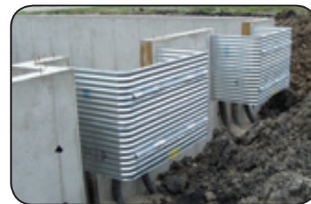
Window wells are connected to the drain tile system.
