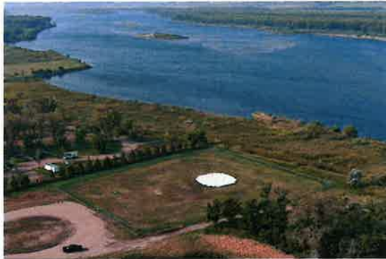
COMPLETED MISSOURI RIVER INTAKE
