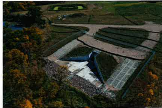
COMPLETED SHEYENNE RIVER DISCHARGE
