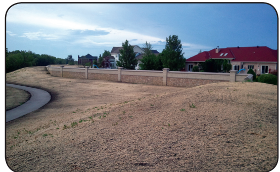
This floodwall in Timberline was recently constructed as part of the City of Fargo's extensive in town flood protection effort. Read more on page 2.
