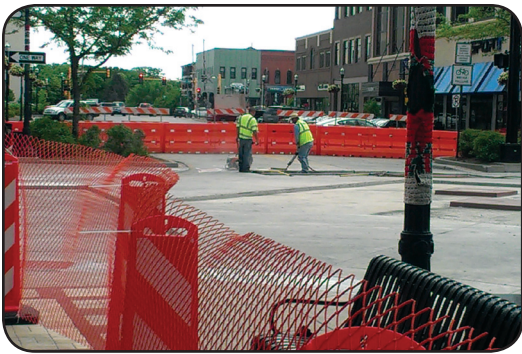
Crews remove and replace deteriorating brickwork at Broadway and NP Avenue.
