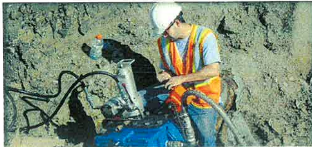
“EZ Valve” Installation
