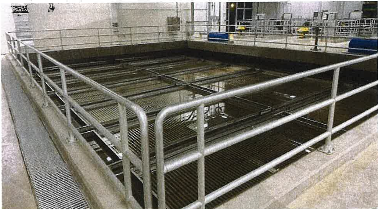
Pretreatment plate settling system in the Membrane Water Treatment Plant (MWTP). The MWTP sludge is high in organic content and more difficult to dewater compared to lime sludge.
