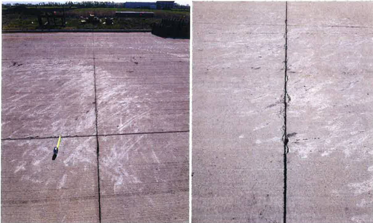
Images show some of the damage from crane
