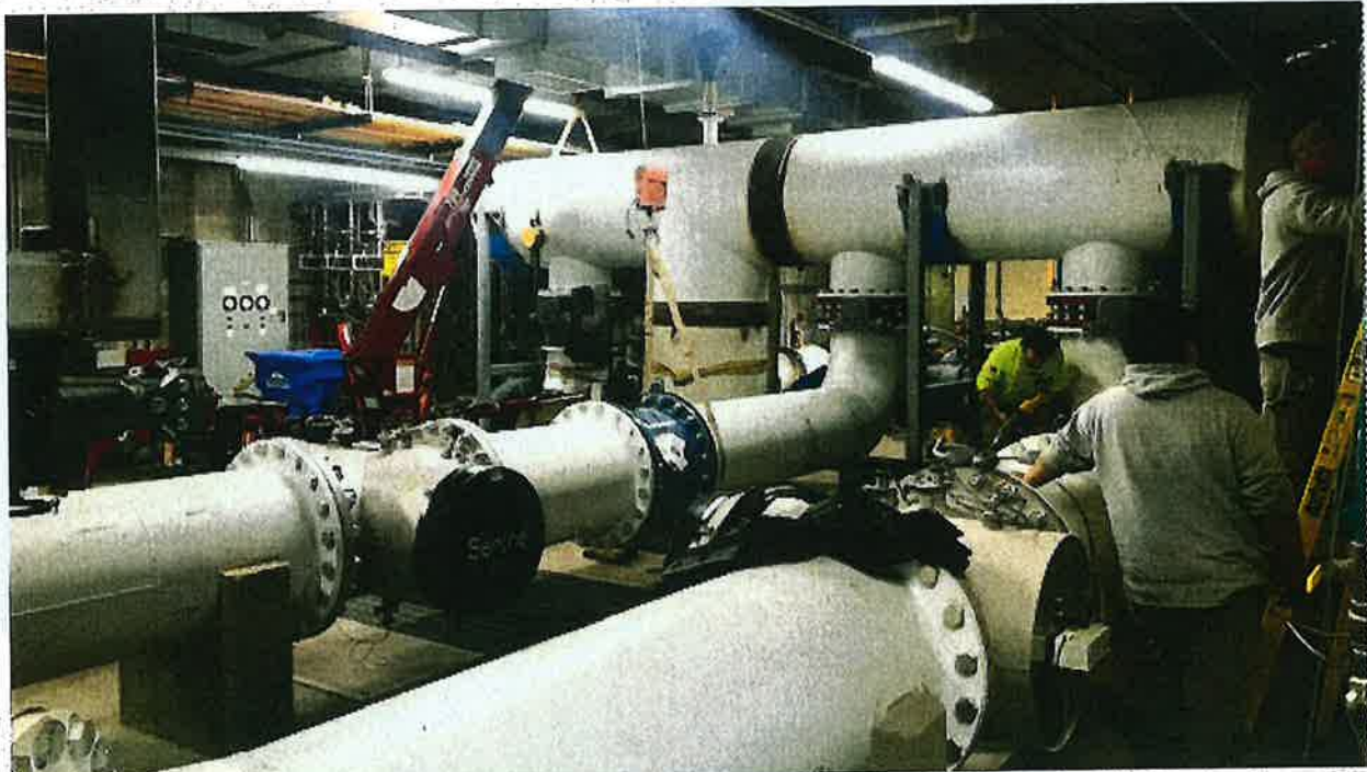
Installation of Ultraviolet (UV) Reactor equipment and piping. Welding, pipefitting, and concrete work required a 6-day shutdown of the 1997 Lime Softening WTP.
