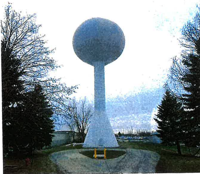
Water Tower #6 (32 nd Ave South)
