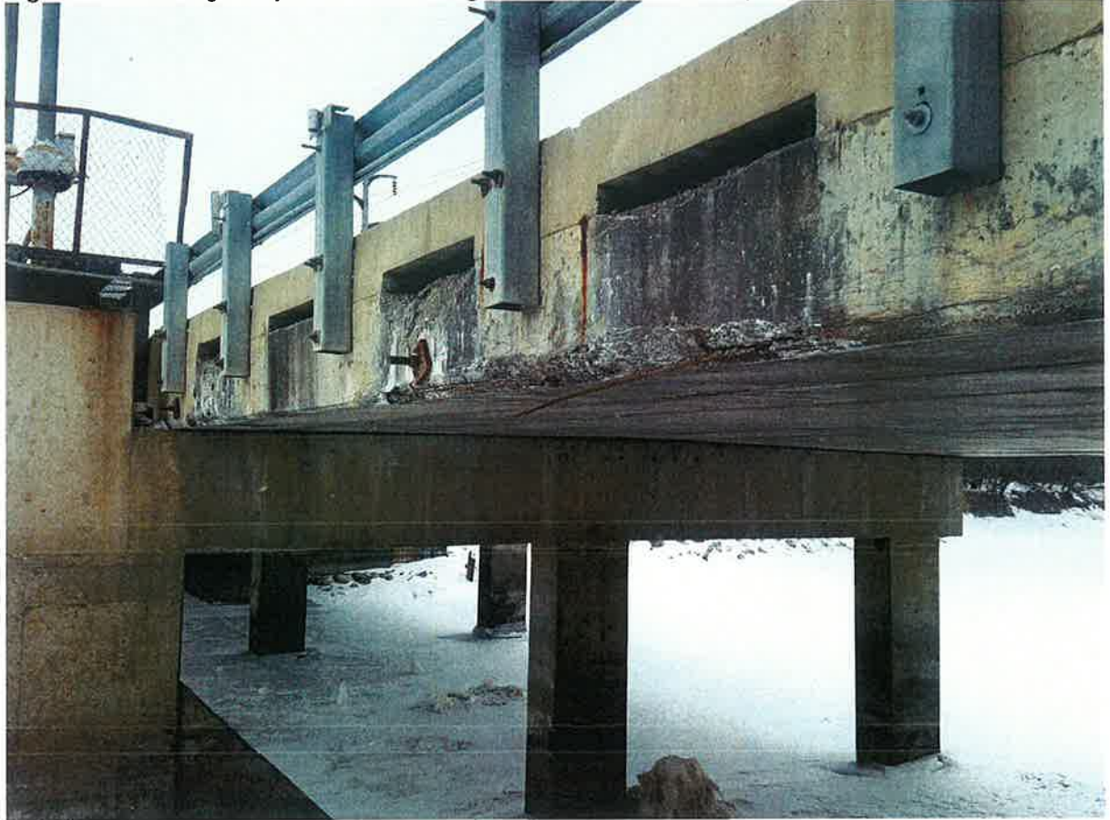
Figure 5 – Existing Sheyenne River Bridge Exterior Beam Damage
