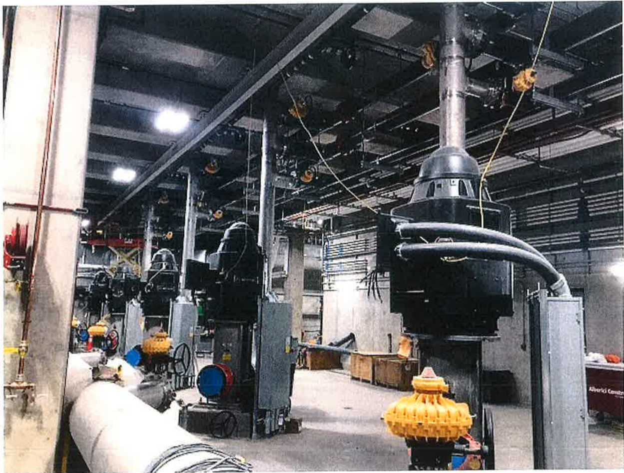
Pneumatic (air-operated) valve actuators - in yellow - for the Reverse Osmosis feed pumps and cleaning systems. Air supply lines will be added to pneumatic valves through-out the MWTP as a change order. Photo from February 23, 2018.
