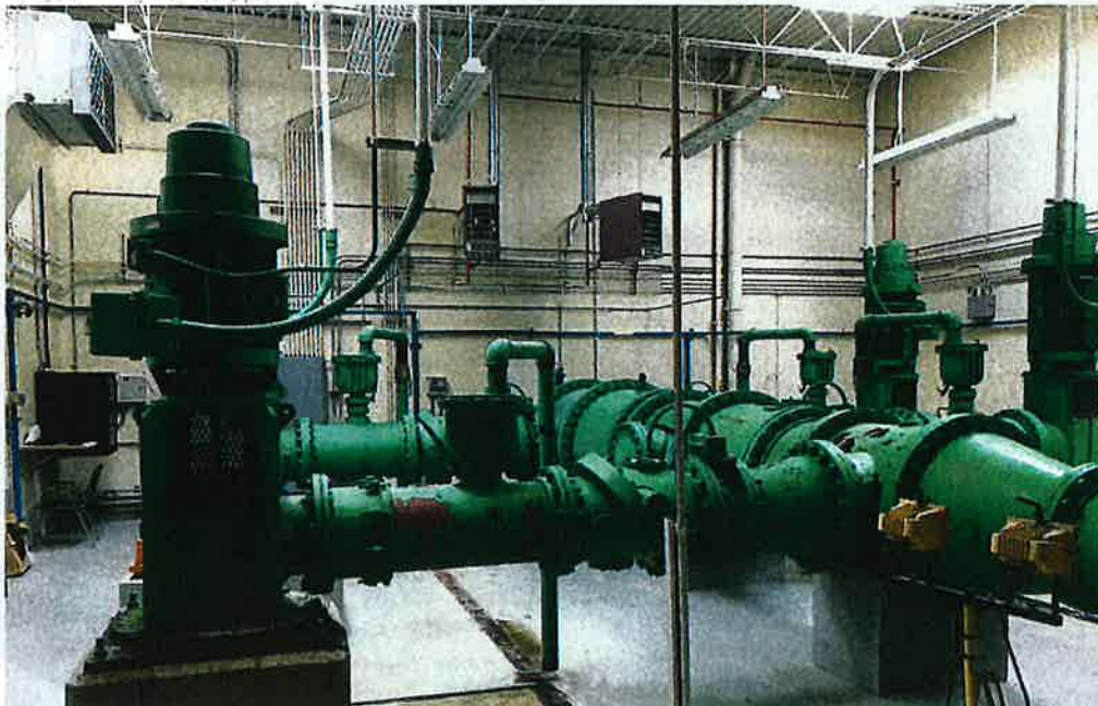
Pumping floor of the Red River Pump Station. This equipment will be replaced or retrofitted to match the current Water Treatment Plant capacity and be raised for flood protection.
