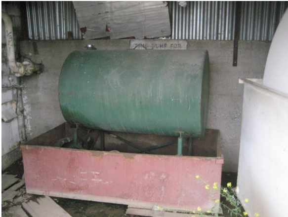
Photo #13 1,000-Gallon Fuel Oil AST Near Boiler Room
