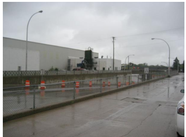
Photo #34 Adjacent Property to the West
