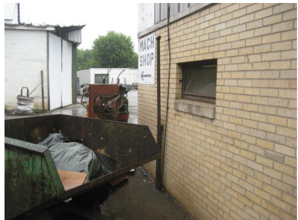
Photo #22 UST Fill and Vent Pile at Northeast Corner of Structural Steel Fabrication Shop #2
