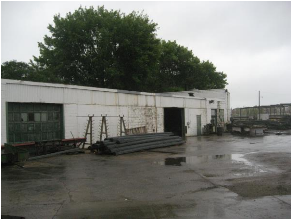
Photo #7 Storage Building
