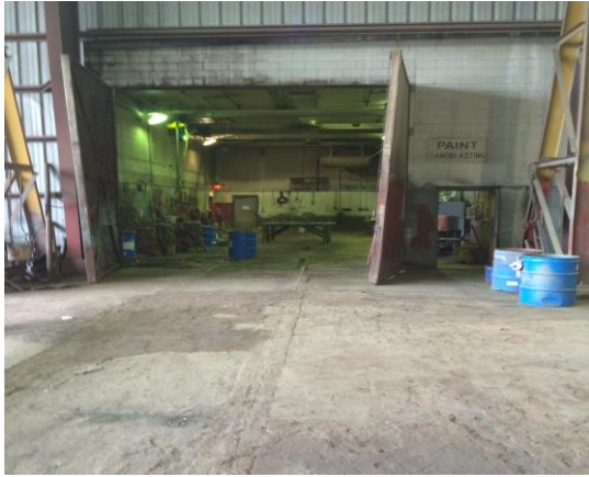
Photo #25 Paint Shop
