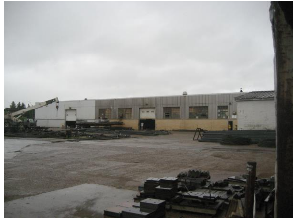
Photo #8 Structural Steel Fabrication Shop #1
