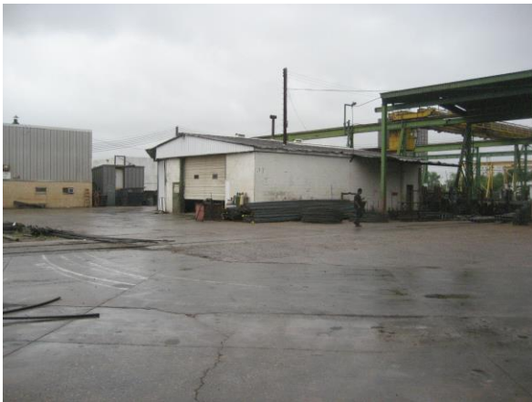
Photo #9 Reinforcing Steel Fabrication Shop
