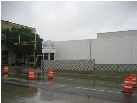
Photo #1 Mid American Steel Looking East
