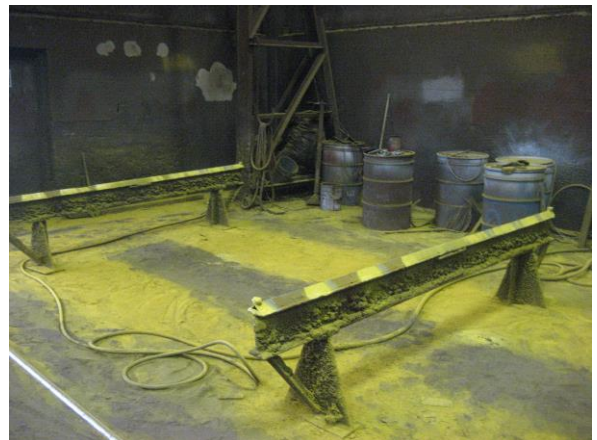
Photo #18 Painting Operations Inside Structural Steel Fabrication Shop #2
