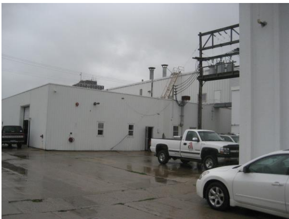
Photo #33 Adjacent Property to the West
