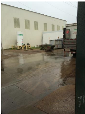
Photo #35 Raw Material Storage Building
