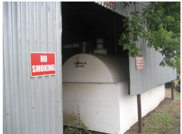
Photo #12 3,000-Gallon Fuel Oil AST Near Boiler Room
