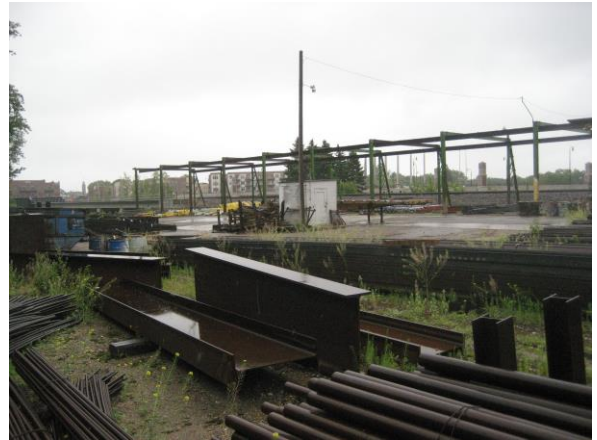
Photo #14 Raw Material Laydown Yard and Weight Scale House
