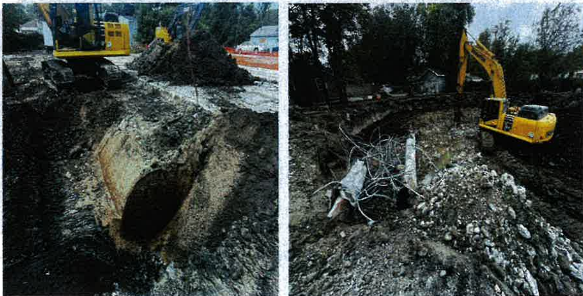
Contaminated Soil Tower #3
