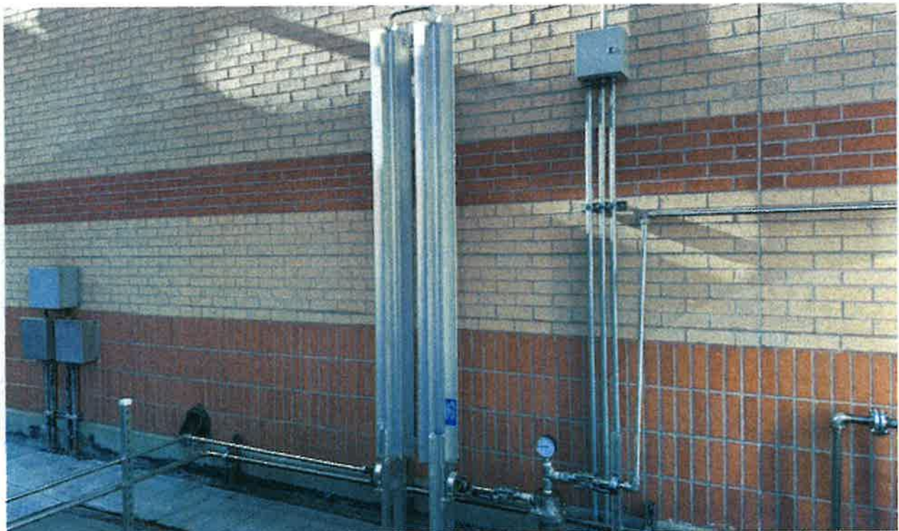
Pictured is some of piping and equipment installed by a specialty contractor to vent Liquid Oxygen (LOX) tank pressure for use in ozone generation (treatment cost efficiency). Apex needs to generate drawings for the North Dakota Department of Environmental Quality (NDDEQ).
