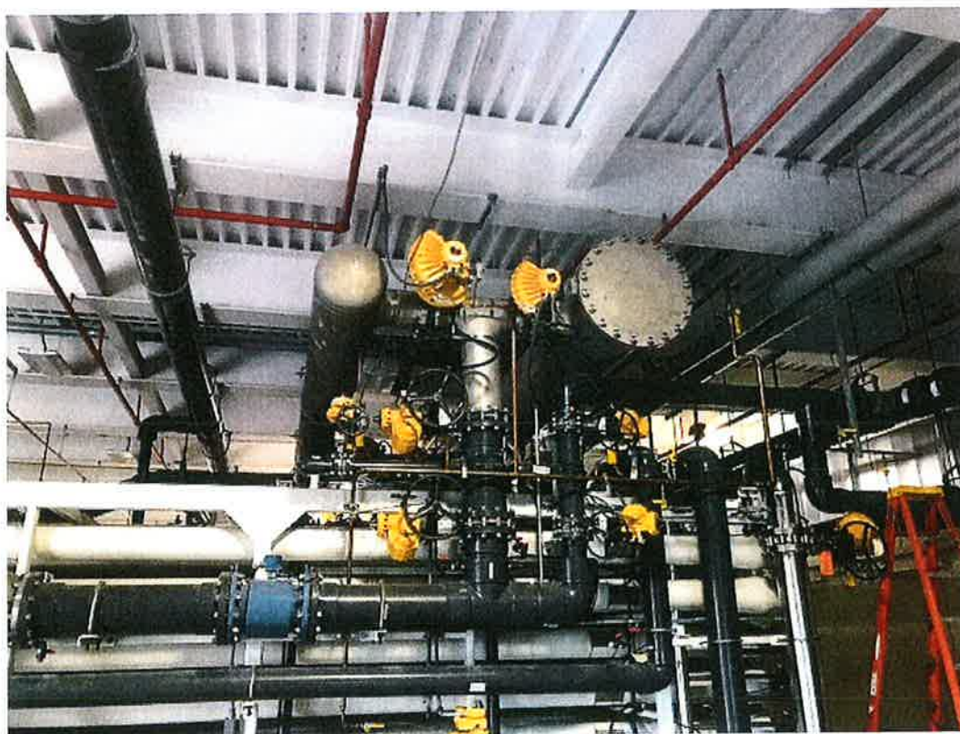
Piping, valves, pressure vessels, and other components on Reverse Osmosis (RO) skid. The RO system has two discharge headers (shown on top) to send RO water to the end of the MWTP or to softening trains in the existing water plant. Photo from June 2018.
