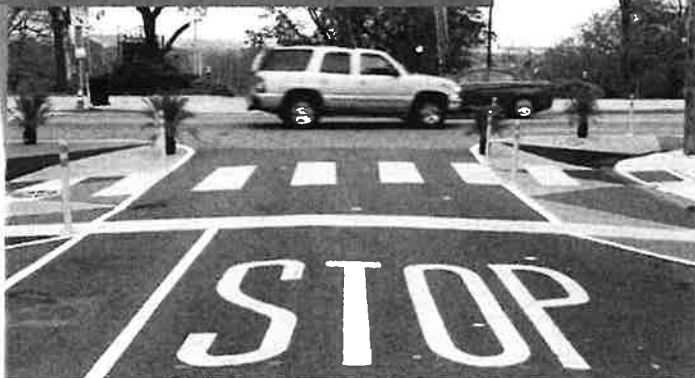
Painted Curb Extensions, Bayside Park, Jersey City
