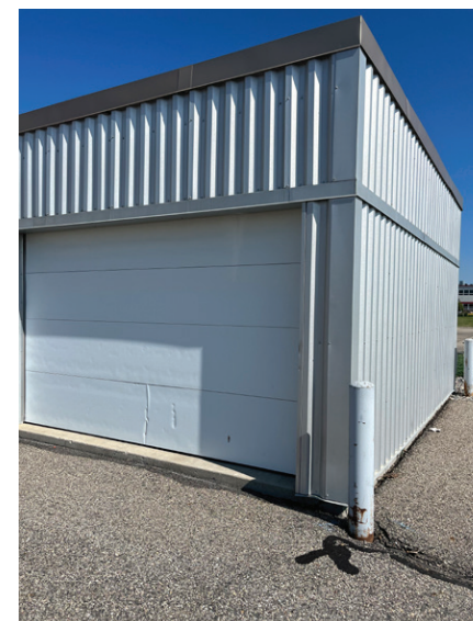
Hazmat Storage Building
