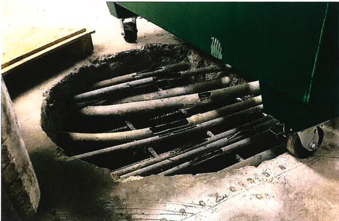
Concrete has been chipped away from conduits in X-ray area. Wires are being traced and will be rerouted to eliminate the pipe route conflict. Piping for the Ultraviolet (UV) treatment system will pass through here.
