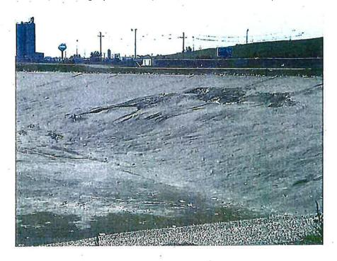
It is imperative that the slope be repaired prior to harsh winter conditions setting so operations can continue unhindered into winter and to preserve the integrity of the remaining liner system in place. The repair work would entail:
