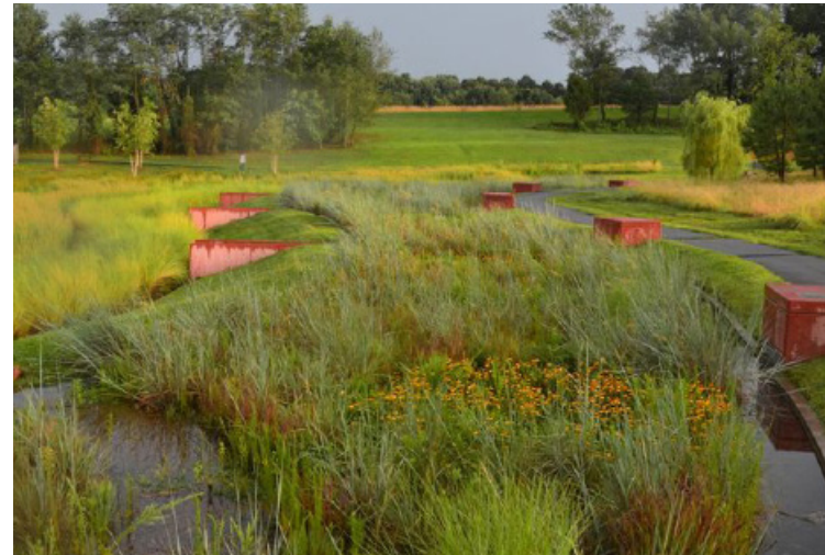
NC Museum of Art Pond Project - stormwater runoff into bioretention terraces and wetland Image Source: https://www.pinterest.com/pin/103231016433542317/
