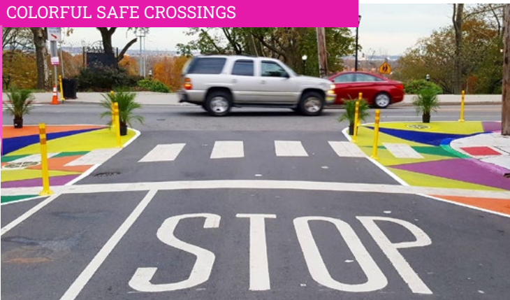
Painted Curb Extensions, Bayside Park, Jersey City
