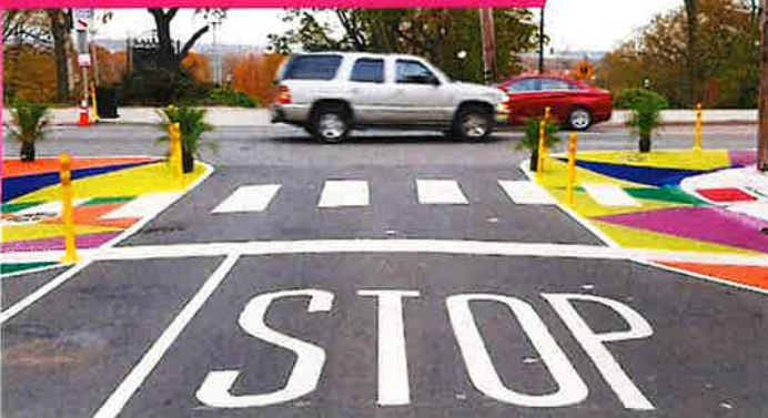
Painted Curb Extensions, Bayside Park, Jersey City
