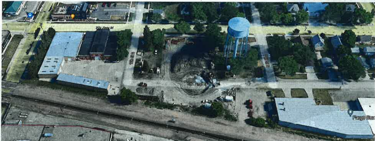
Construction site for new Downtown Water Tower and location of existing Water Tower #1.
