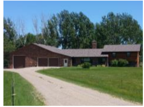
Neighboring Property across the street to the East
