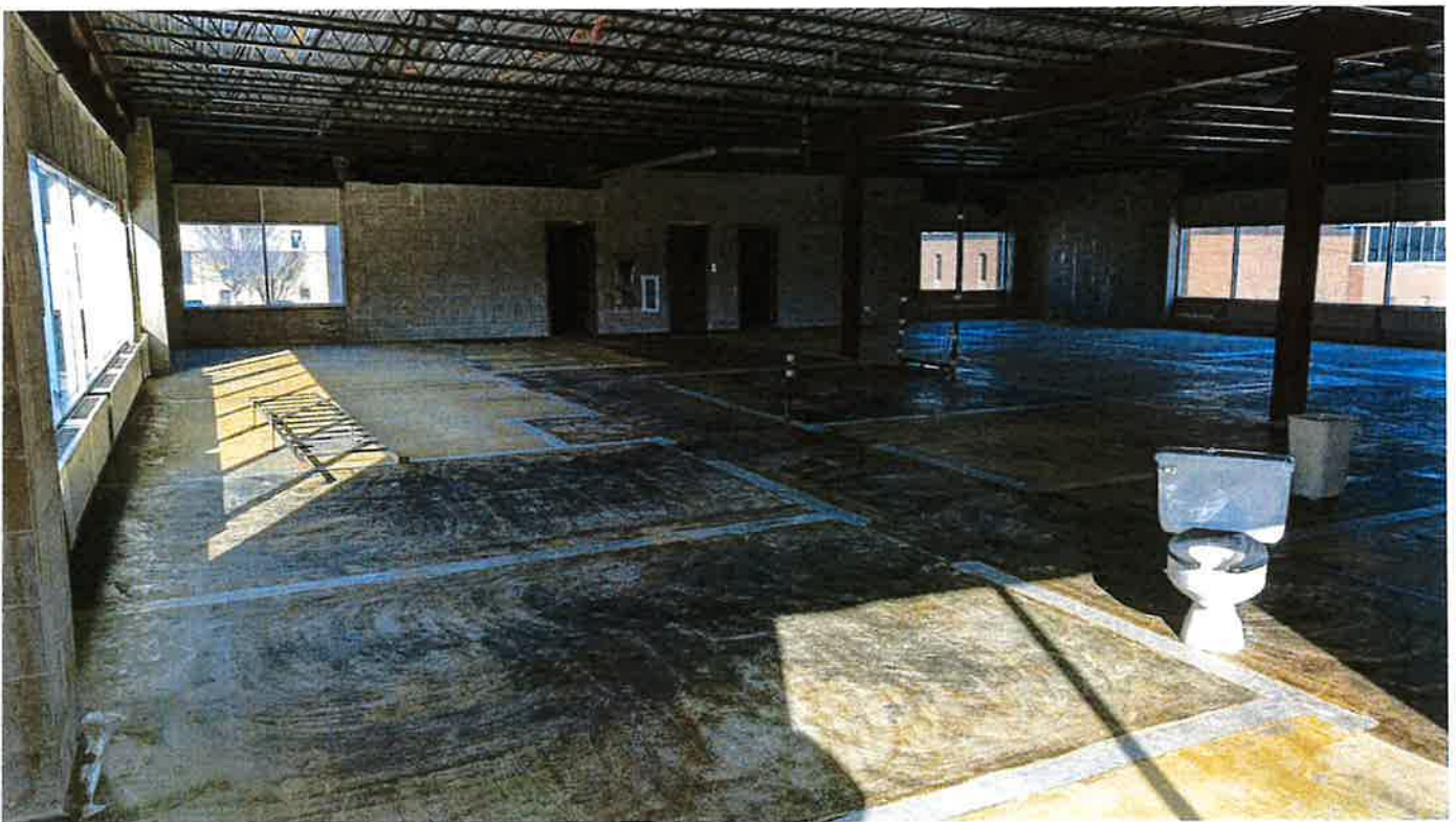
Images of interior after asbestos abatement
