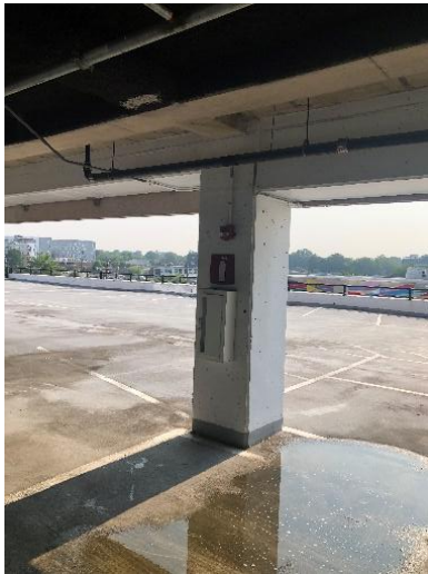
Figure 19 - Ponding Water
