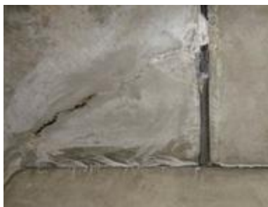
Figure 8 – Leaching Concrete
