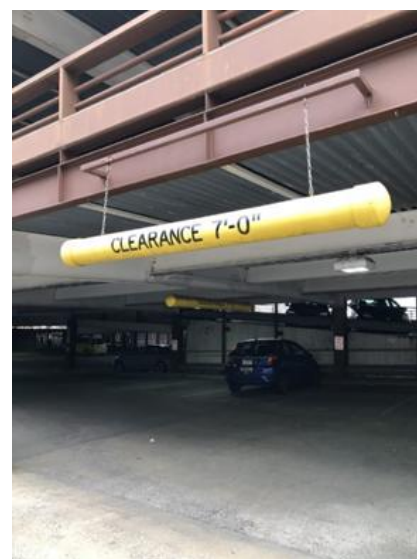
Figure 35 - Typical Headache Bar
