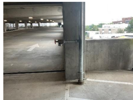
Figure 26 - Typical Fire Department Connection
