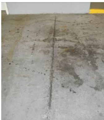
Figure 13 – Typical Construction Joint
