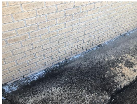
Figure 16 - Stain Buildup
