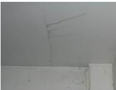
Figure 7 – Leaking Crack
