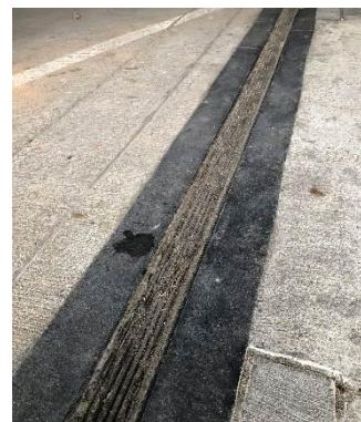
Figure 15 – Typical Winged Expansion Joint
