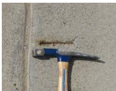
Figure 12 - Exposed Reinforcement
