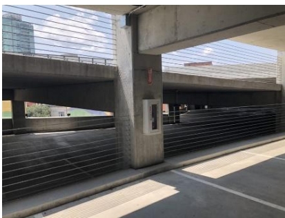
Figure 32 - Typical Barrier Cable
