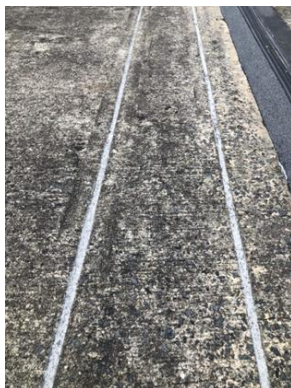
Figure 14 – Typical Joint over Steel Beam
