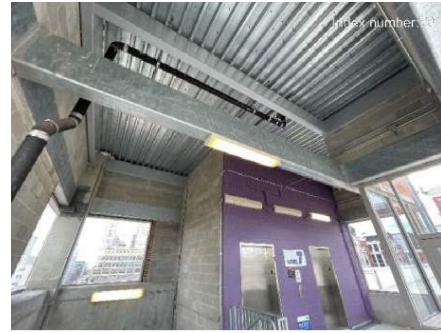
Figure 24 - Elevator at River South (photo courtesy of the 2022 SC Condition Assessment Fluorescent Light Fixture)
