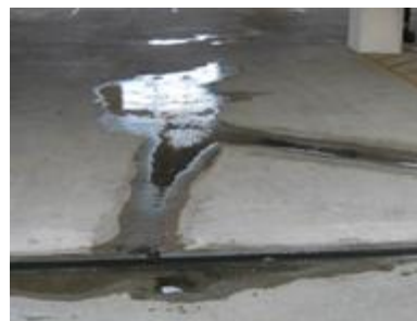
Figure 9 – Ponding Water
