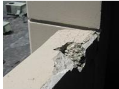
Figure 3 - Concrete Spall
