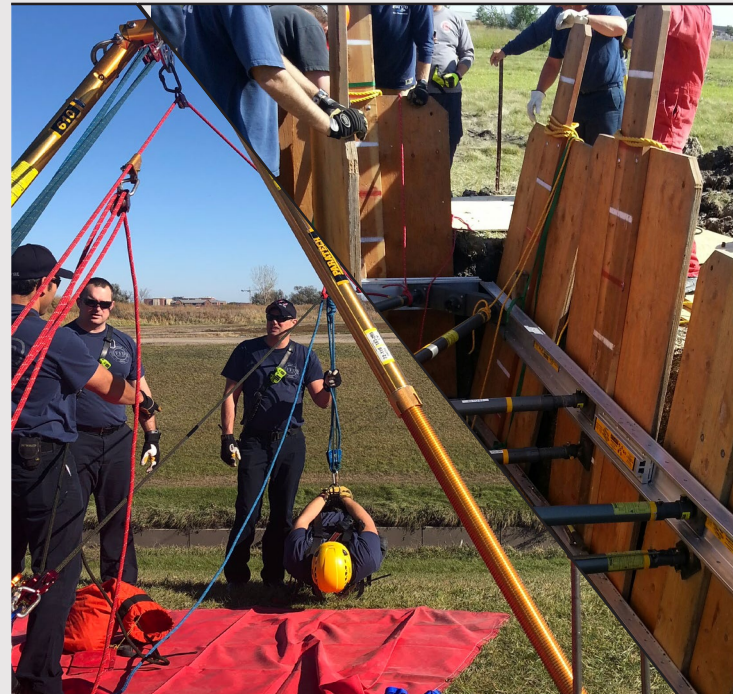
Tripod set up to lower and raise rescuers and victims
