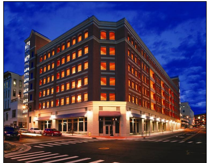
Figure 21 Monroe Center Parking Structure
