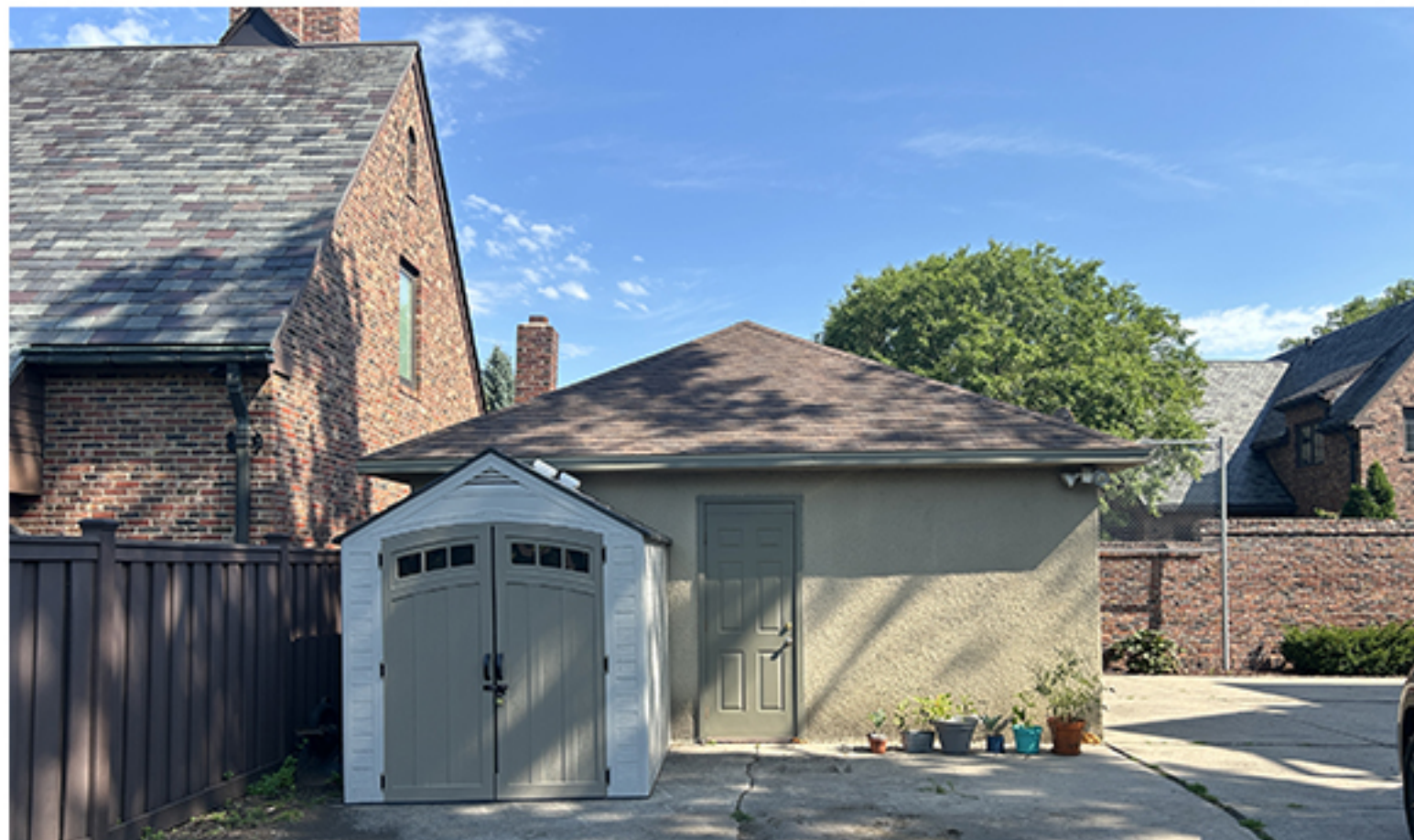
Exterior View - South
