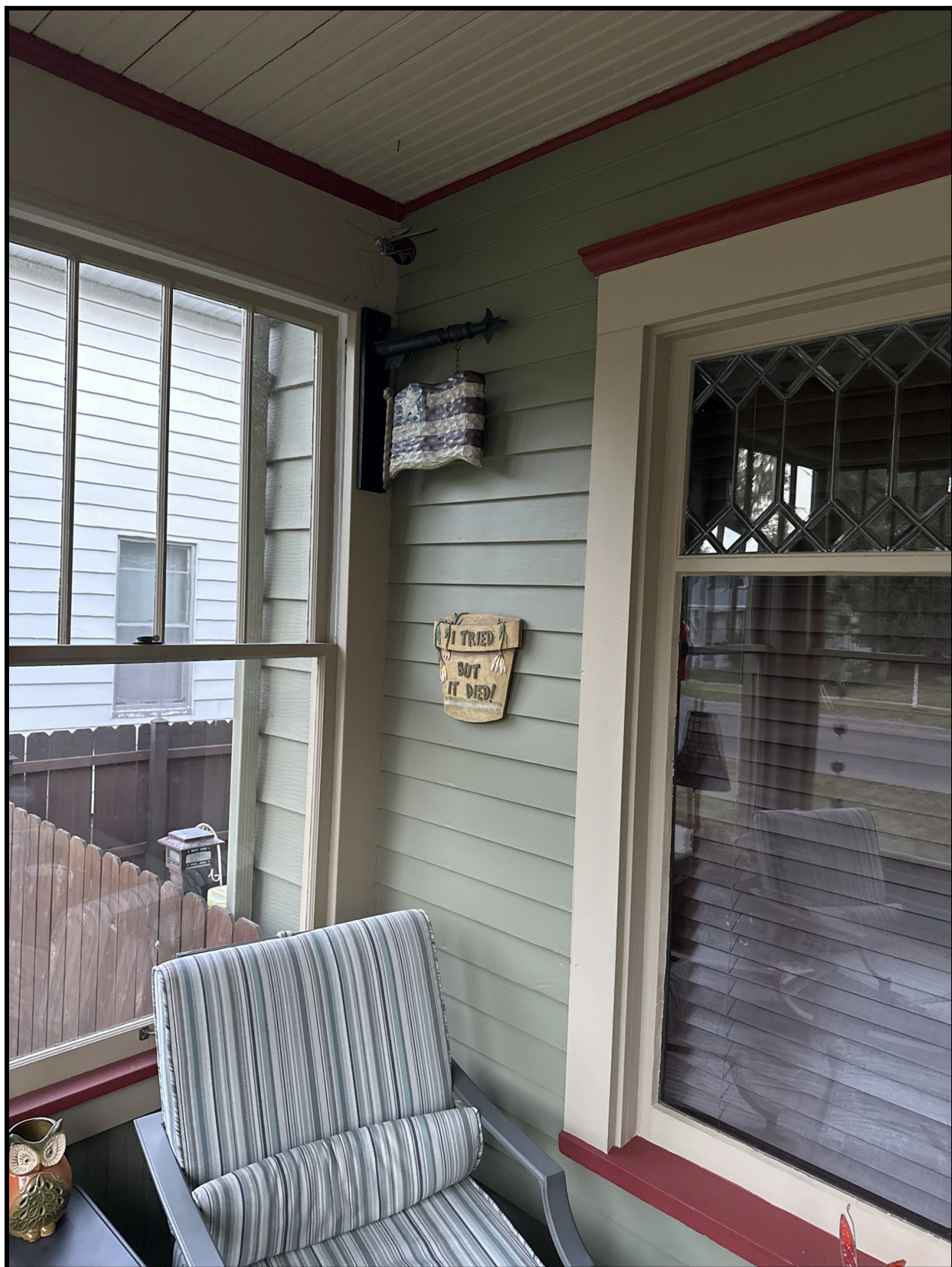
Porch interior on front of house showing existing and original siding:
