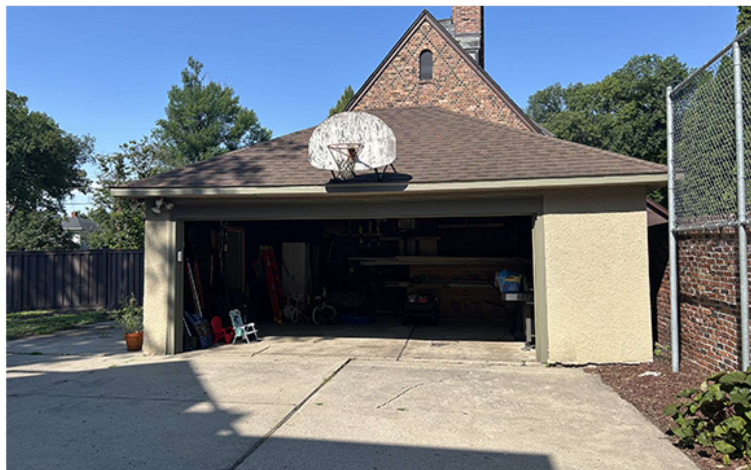
Exterior View - East
