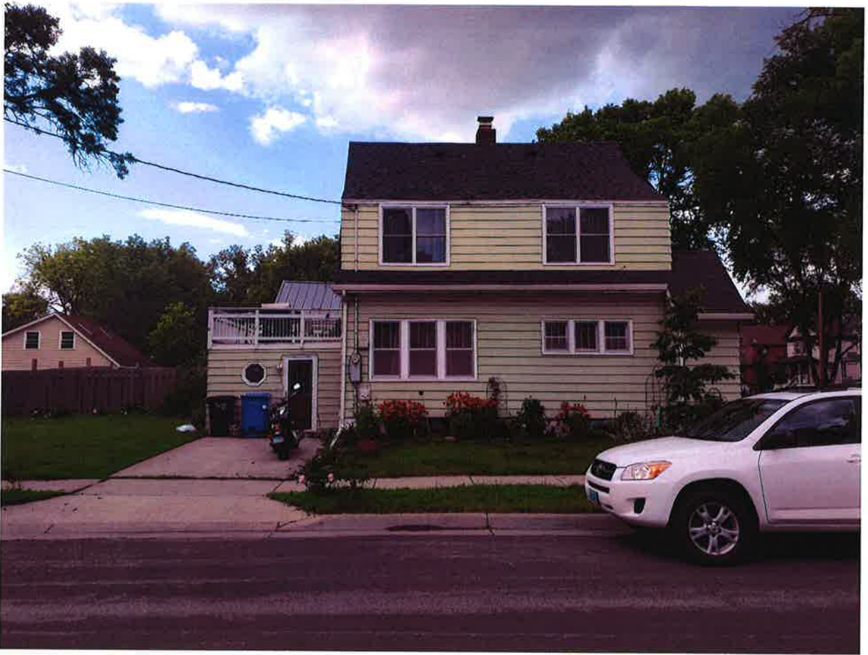
South side of house
