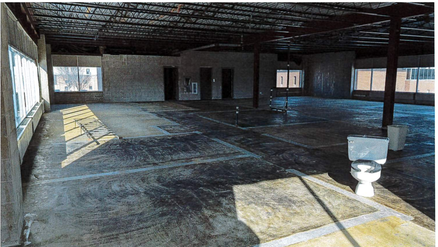
Images of interior after asbestos abatement
