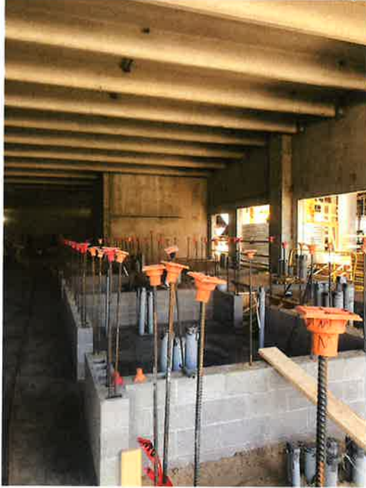
Photo 1 – Ground tier mechanical rooms masonry wall construction in progress.
