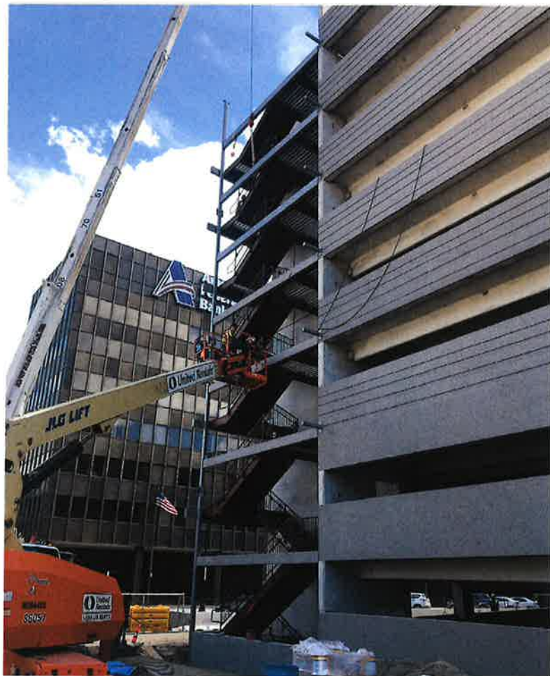
Photo 3 – Northeast stair tower metal stair installation nears topping out. Mobile erection crane working from 3 rd Avenue North
