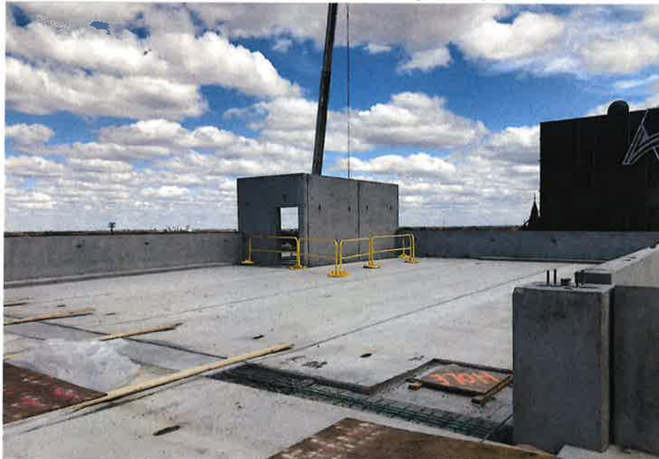
Photo 2 – Parking Garage precast erection complete. Looking north east at north stair tower. Curb and concrete wash installation just beginning from top down.
