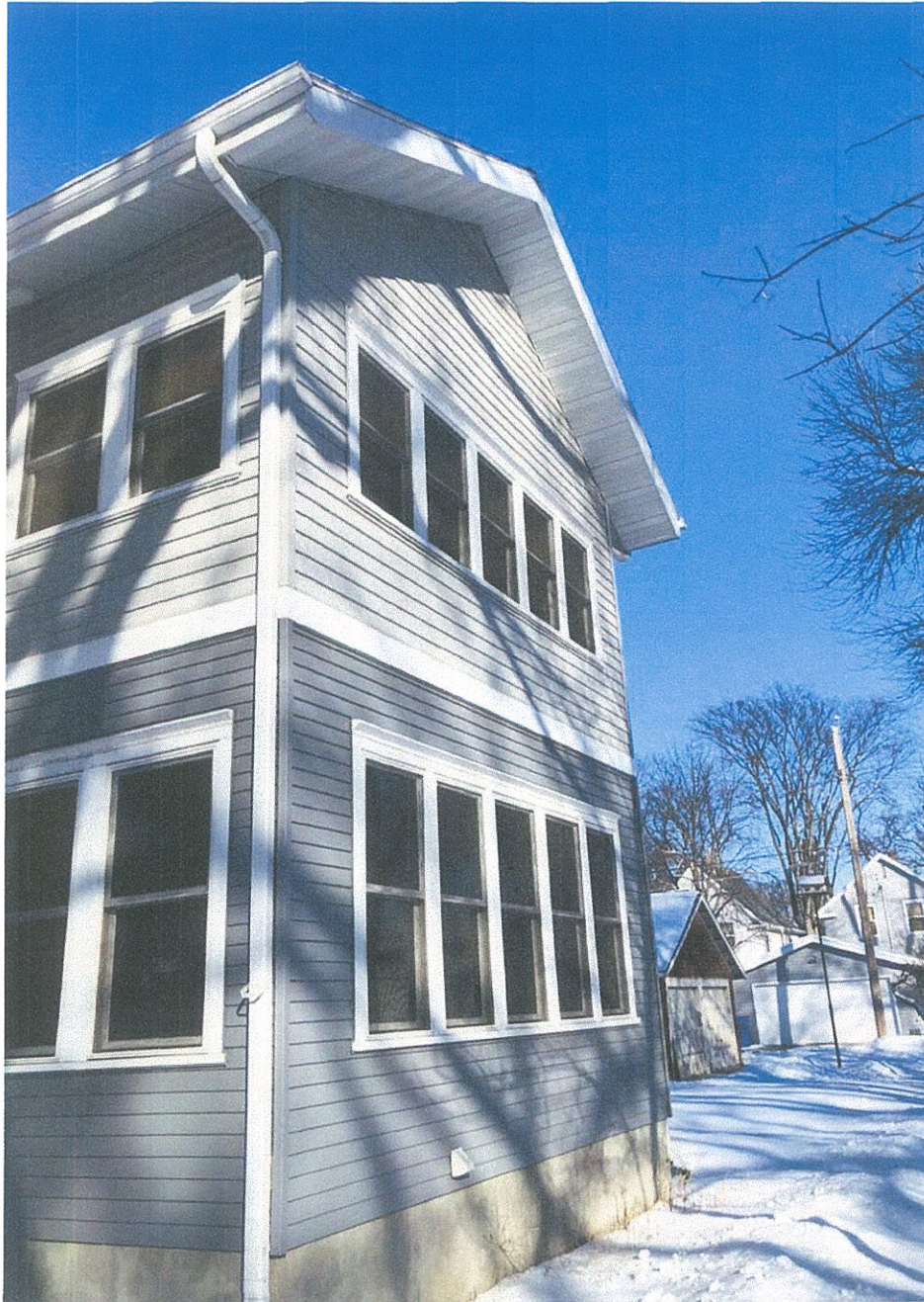
South Elevation (Street Side) of House
