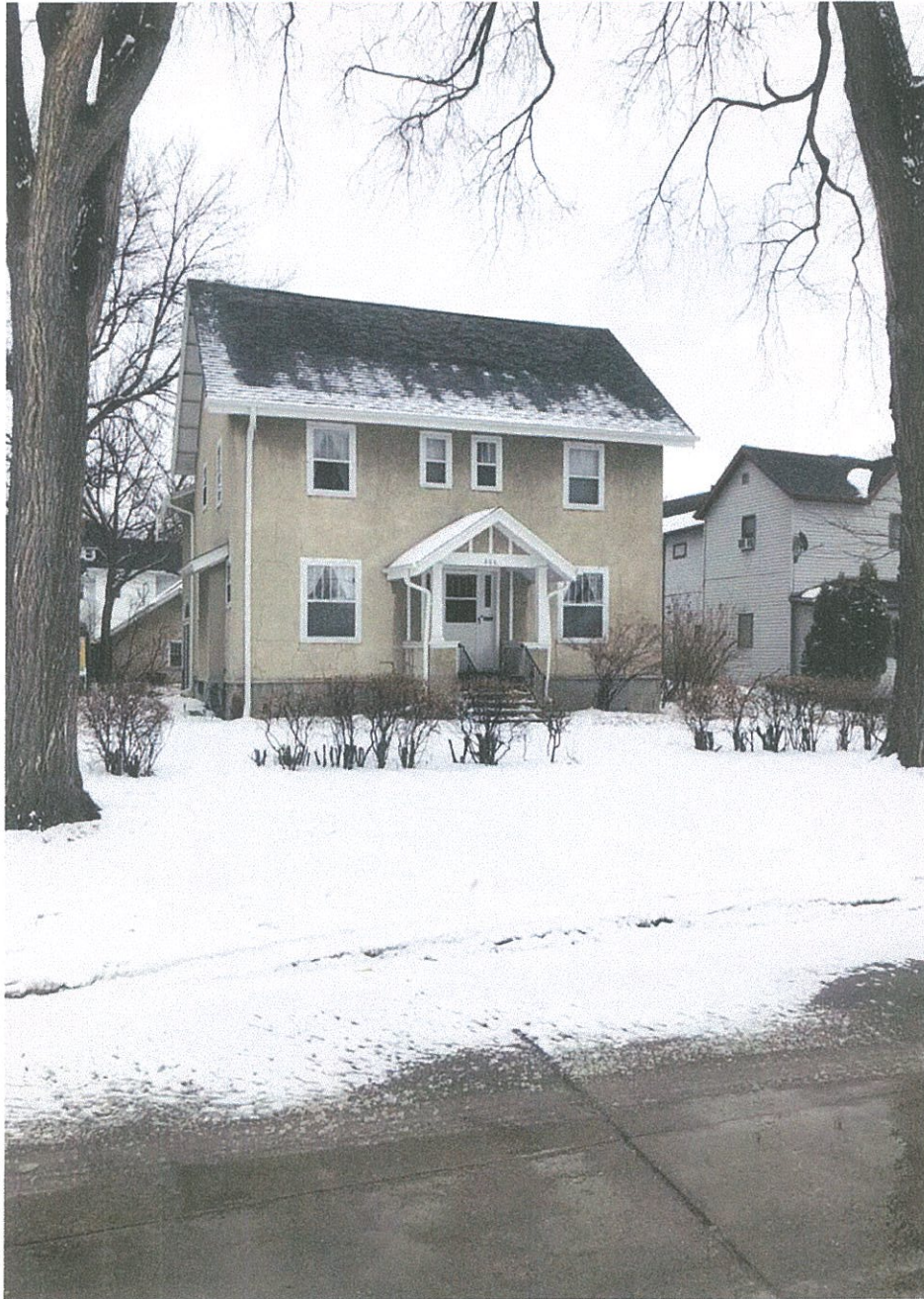
West elevation of house - Front
