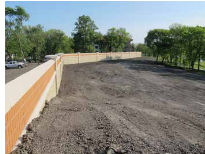
③ Levee and flood wall at 13th Avenue
