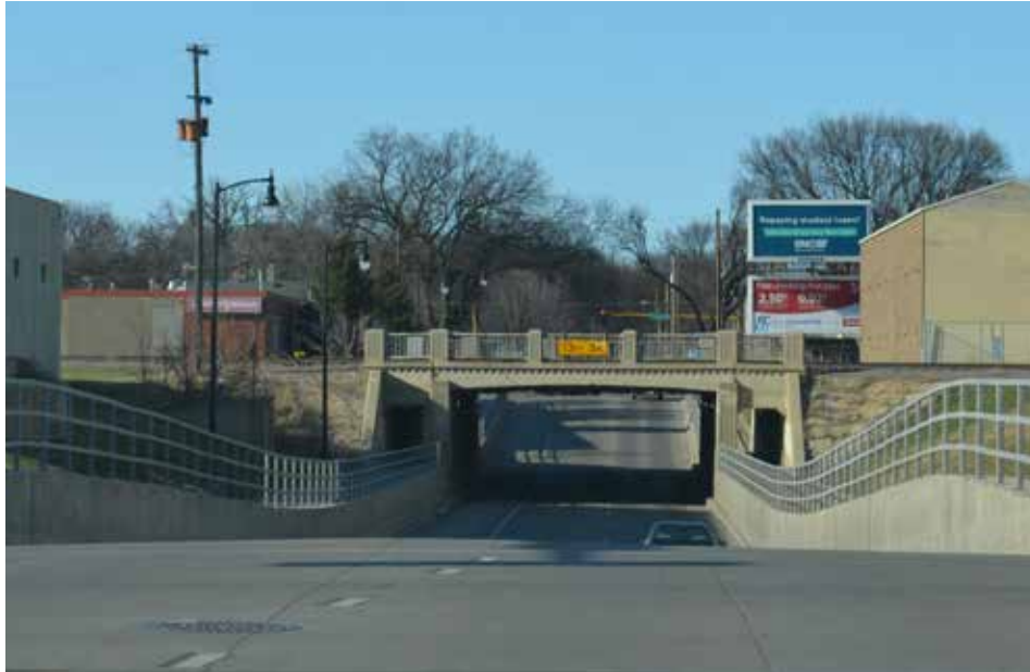
Overpasses and concrete walls
