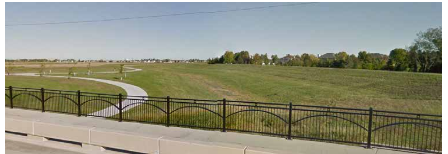
⑤ Bike trail and drainage ditch from 52nd Avenue
