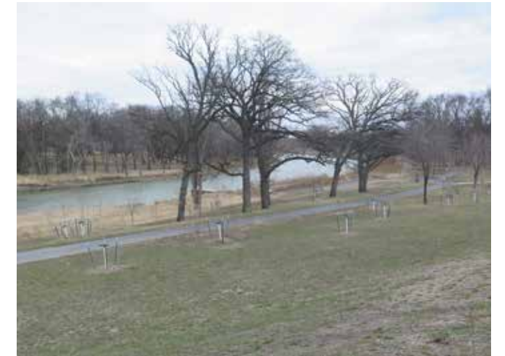
③ Levee and flood wall at 13th Avenue
