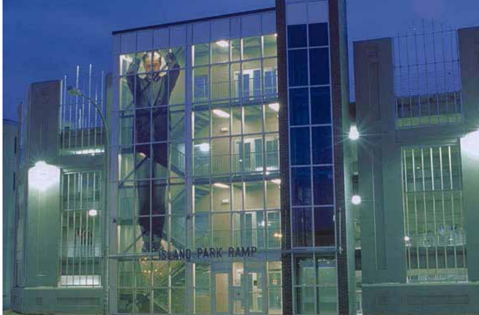
Atlantean - Island Park Ramp
