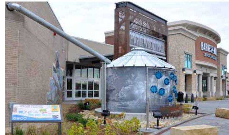
Maplewood Mall interactive stormwater demonstration project. Image Source: http://www.corridorsofopportunity.org/Corridors_News/open-space-public-art-support-stormwater-management
