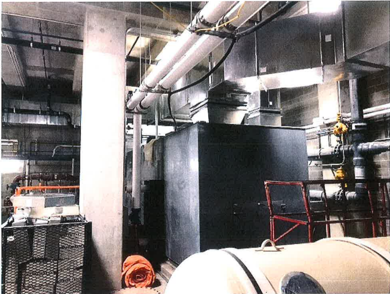
Air Handling Unit in MWTP Lower Level Reverse Osmosis Pump Room. Photo from January 29, 2017.
