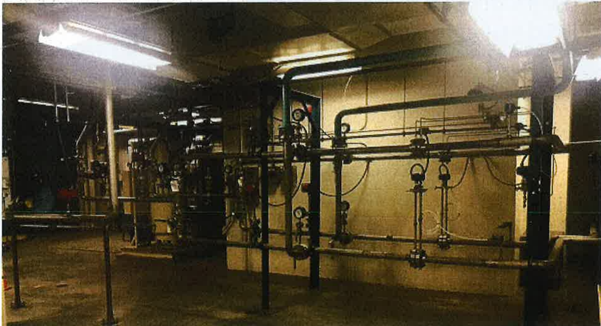
Piping in the ozone generation room. The mixing of ozone with outside air results in nitric acid in downstream piping and corrosion issues where gas interfaces with water.
