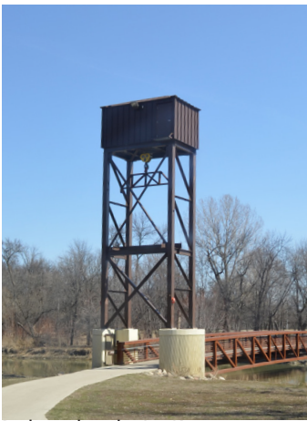
Bridge - photo by Jen Krava
