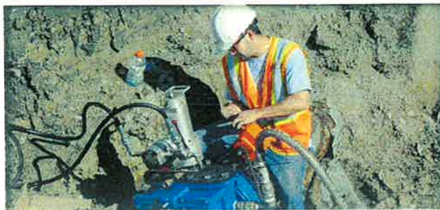
“EZ Valve” Installation
