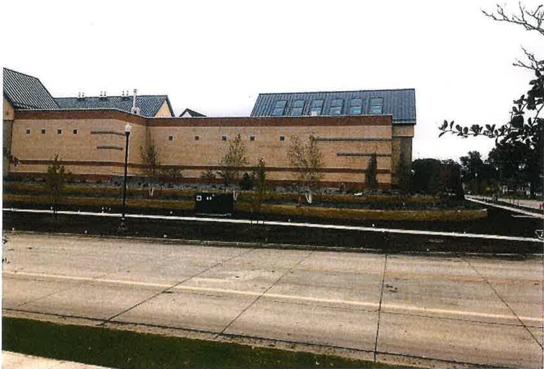
View of MWTP at the corner of 13 th Avenue South and 5 th Street. Retaining block wall and new sidewalk are shown. Photo is from September 29, 2018.
