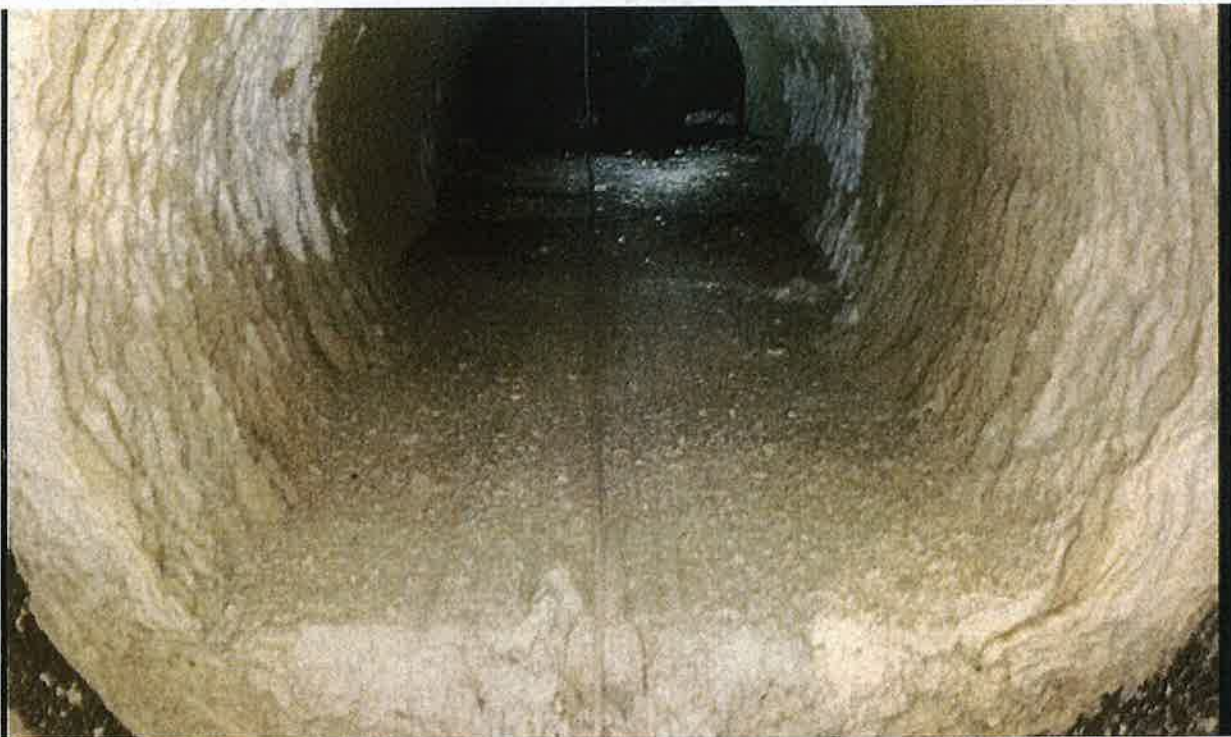
42-inch Pipe showing scale buildup in Softening Train #2. This pipe is deep under the Water Treatment Plant and was cleaned by Hydro Klean this past spring.
