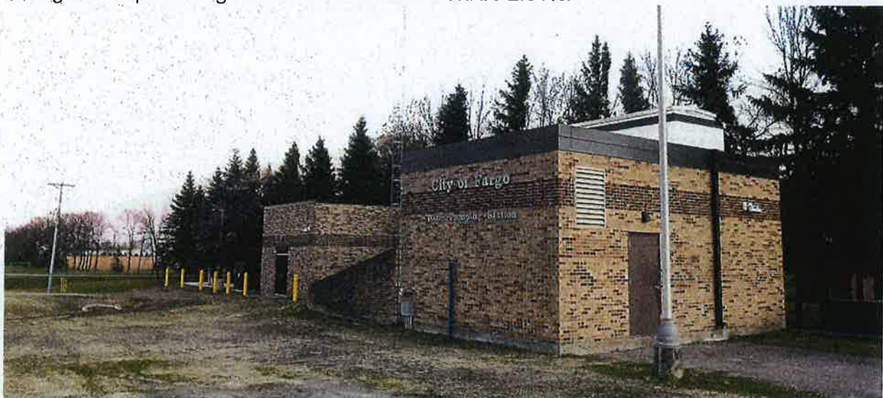
Sheyenne River Pump Station with new electrical building under construction (Summer 2018).
