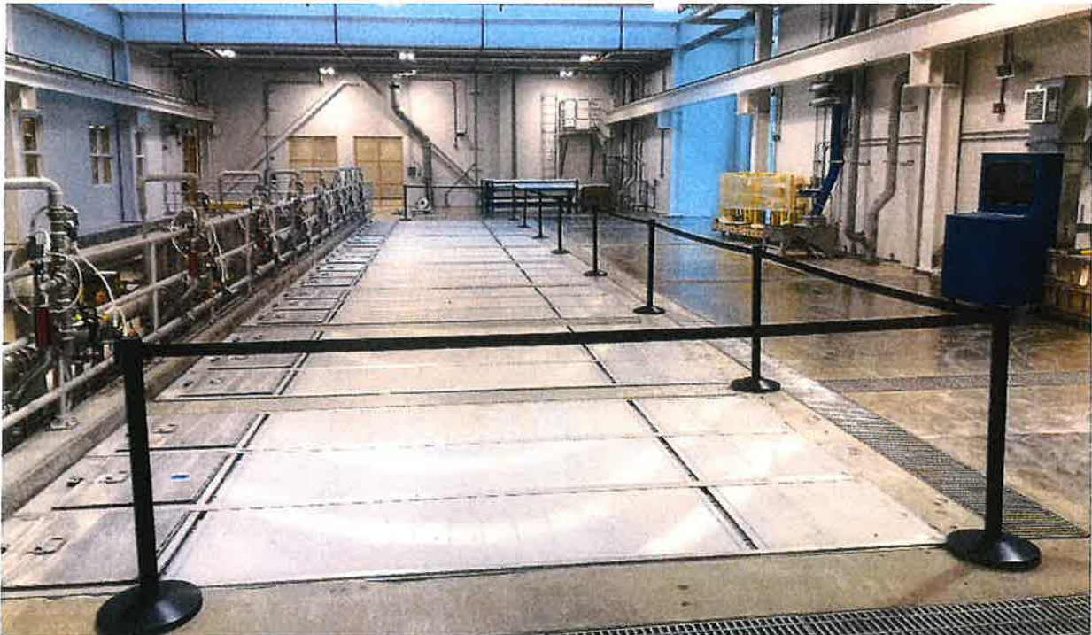
View of Microfiltration/Ultrafiltration room on the main level of the MWTP. Concrete floor is sealed and area has been mostly cleaned up of construction debris. Photo from October 2018.
