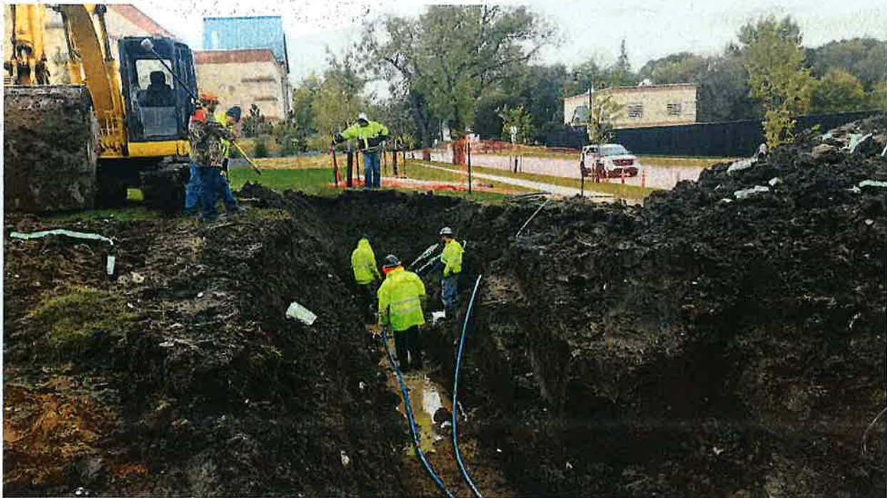
Water sample line modifications has alleviated air issues that resulted in sample pump stoppage and noise interference with instrumentation monitoring EPA-regulated parameters.
