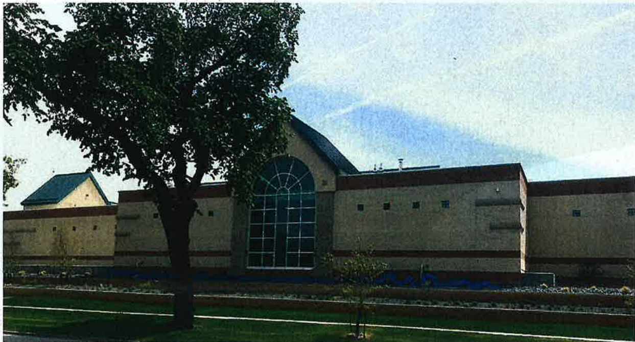
View of the new MWTP from 13 th Avenue South. The MWTP has been fully operational since June, 2019.
