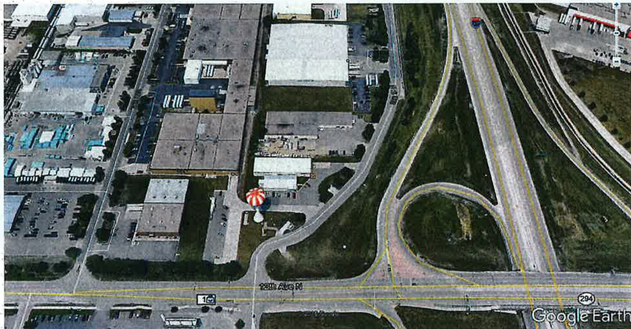
Water Tower 4 in North Fargo has Federal Aviation Administration (FAA) Requirements.
