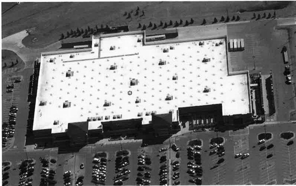
Super Walmart (Front View – Looking East)
