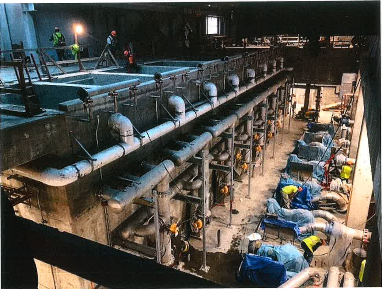
Construction of Ultrafiltration system. General Electric (Suez) is manufacturer. Photo from October 7, 2017.
