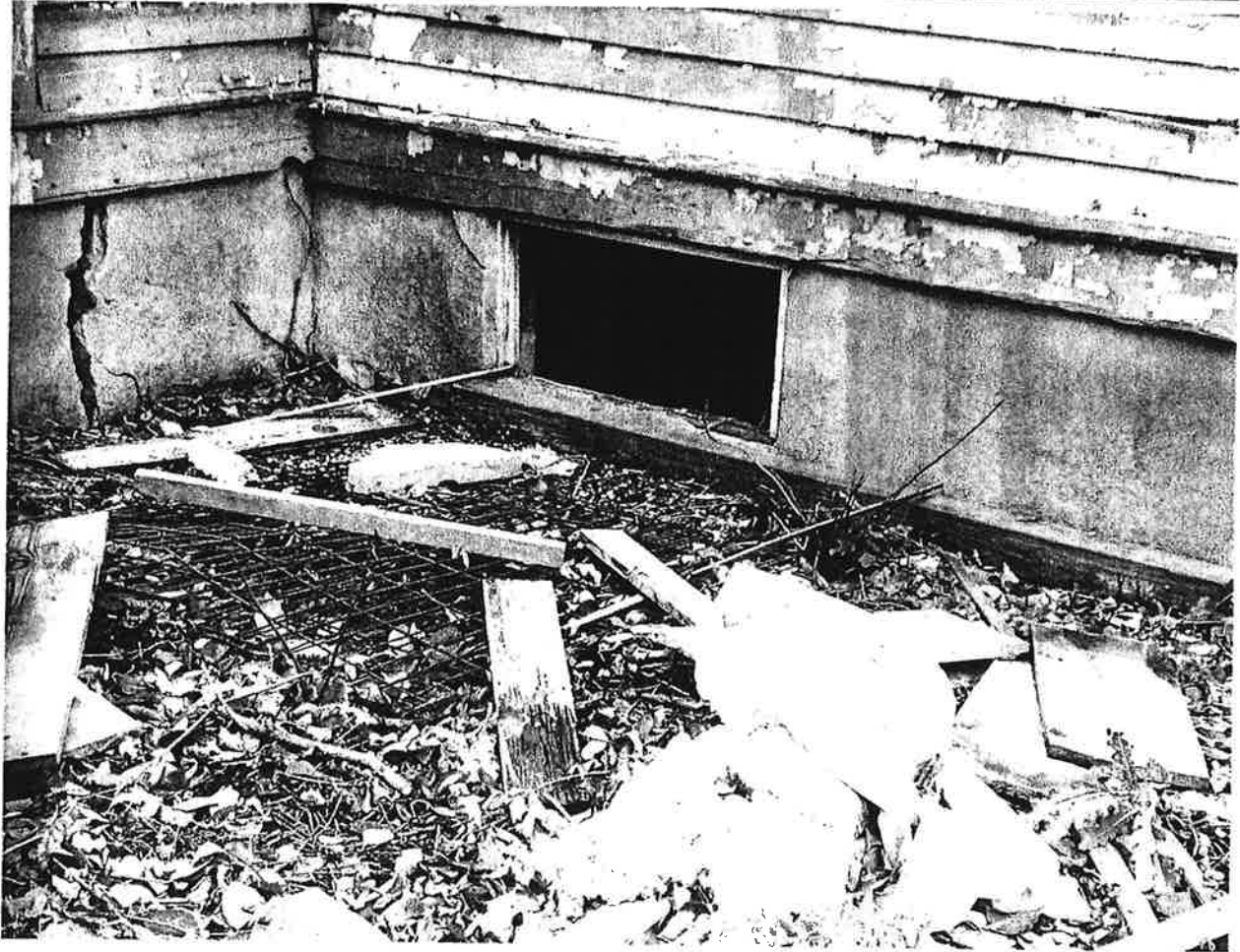
1101 7 Street N., Fargo, ND - 11/1/2018 Unsecured Building
