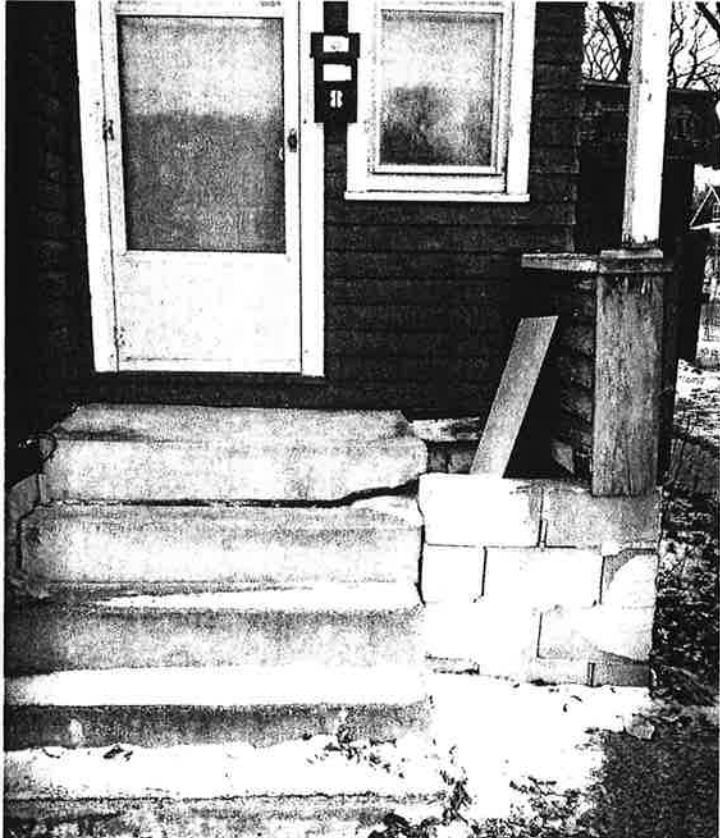
826 10 Street N., Fargo, ND 12/13/17 Unsecure/Unsafe Building Photos
