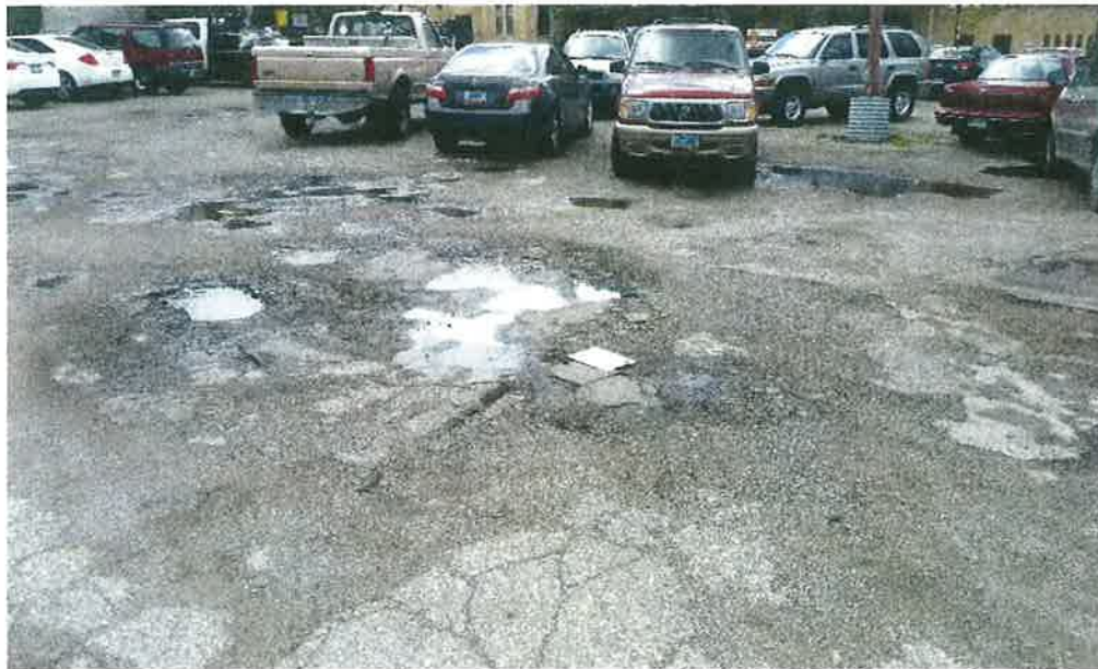
Heartland south parking lot 2016 – asphalt heavily potholed, cracked and patched throughout
