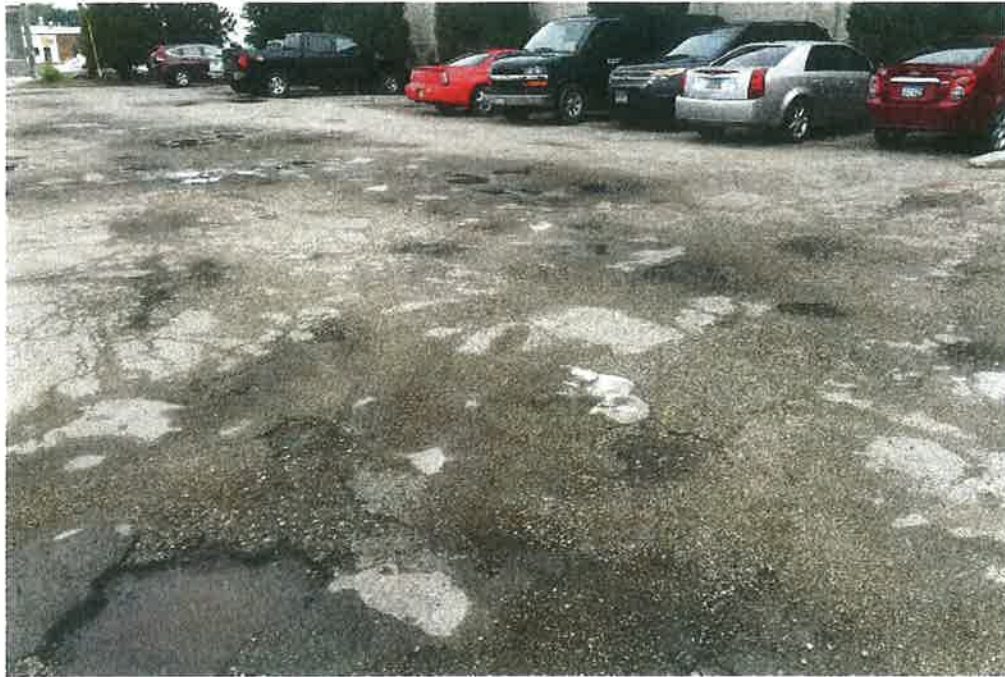
Heartland south parking lot 2016 – asphalt heavily potholed, cracked and patched throughout
