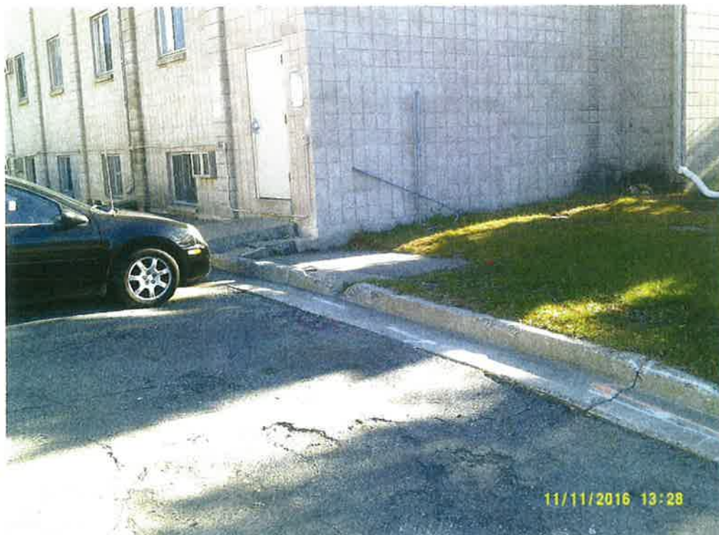
Heartland north parking lot exterior wing entrance – concrete steps and curbing are damaged
