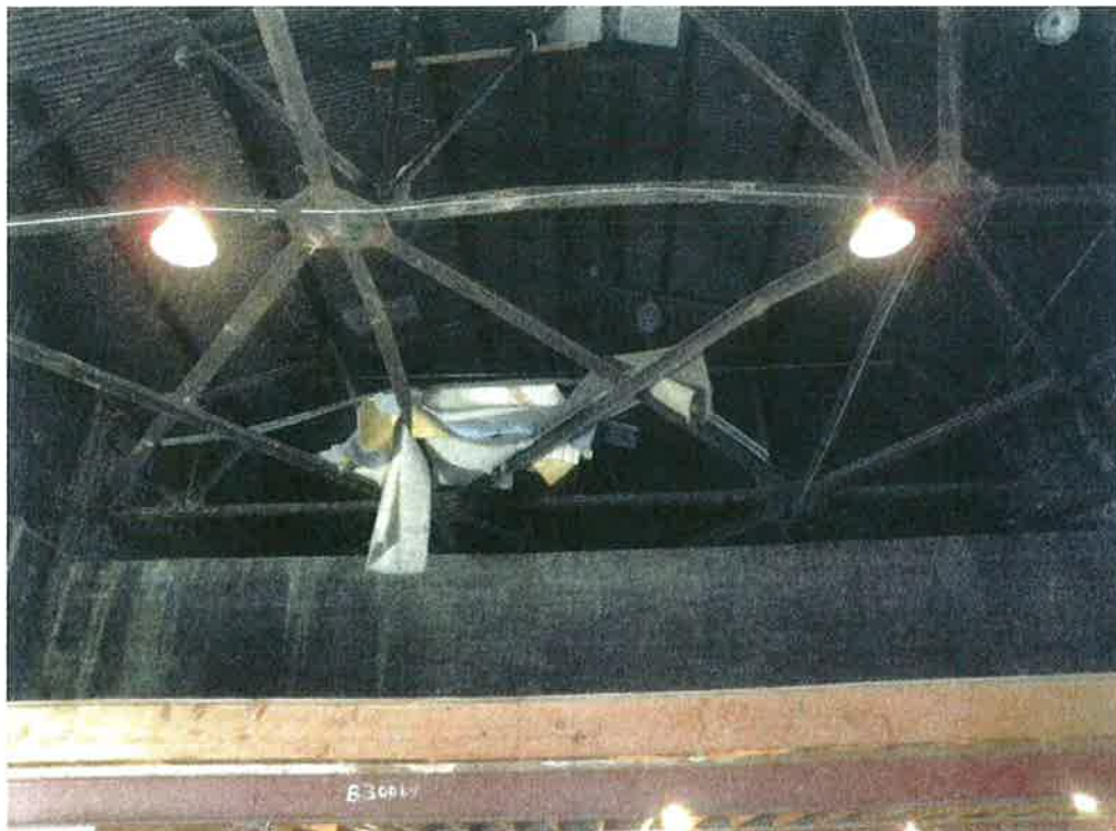
North storage building inside view of ceiling rafters – lead paint on surfaces
