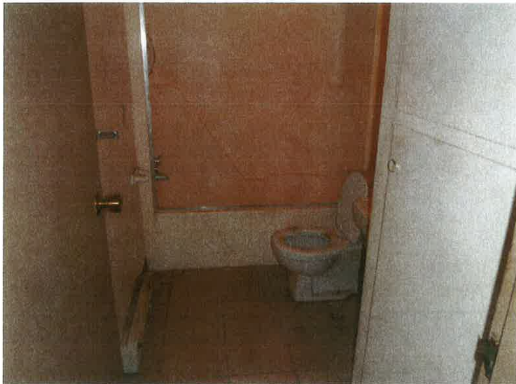
Heartland Building Apartment 10A – bathroom walls/floors stained, overall poor condition
