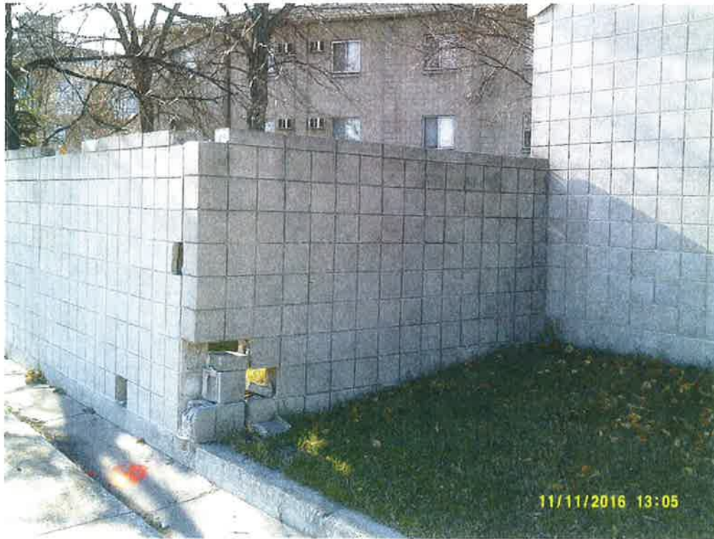
East courtyard wall – numerous blocks are cracked or missing and the wall is overall in poor condition
