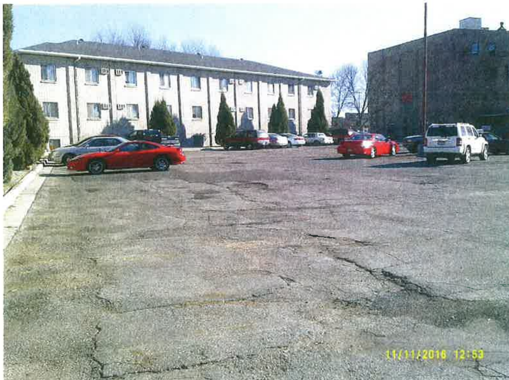
Heartland south parking lot view to the east – asphalt heavily cracked and patched throughout
