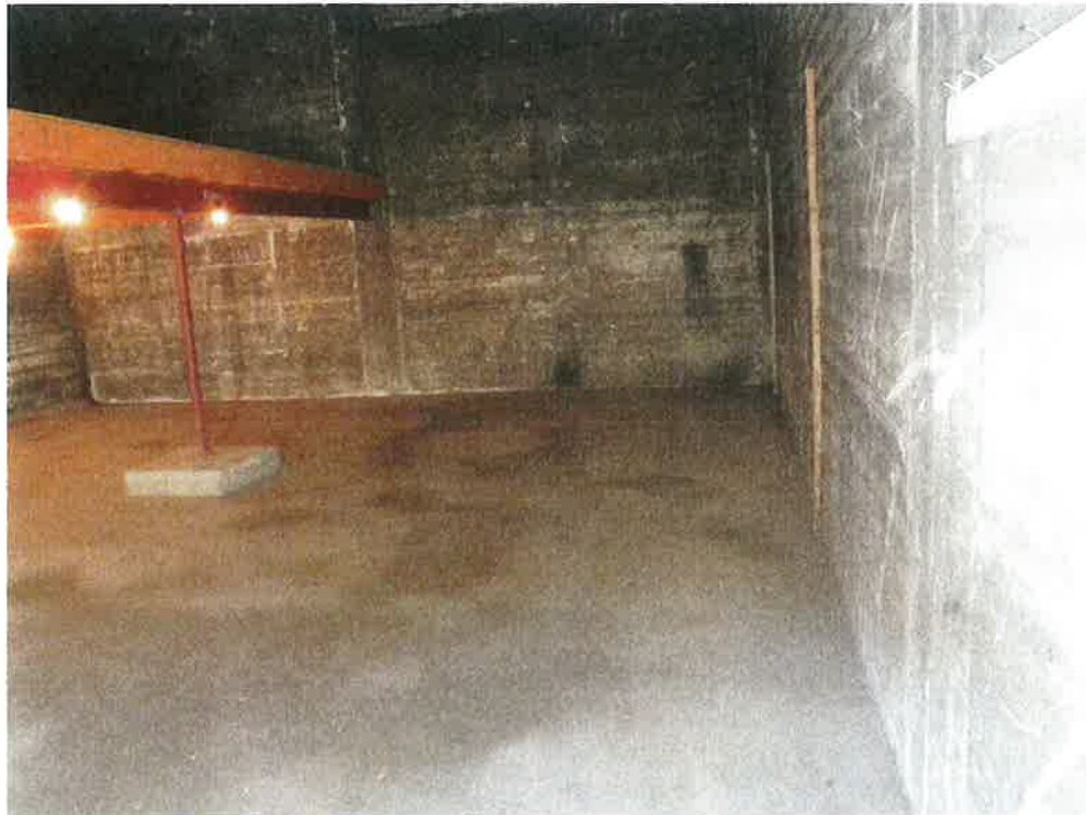
North storage building inside view of east storage area – loft area in upper left
