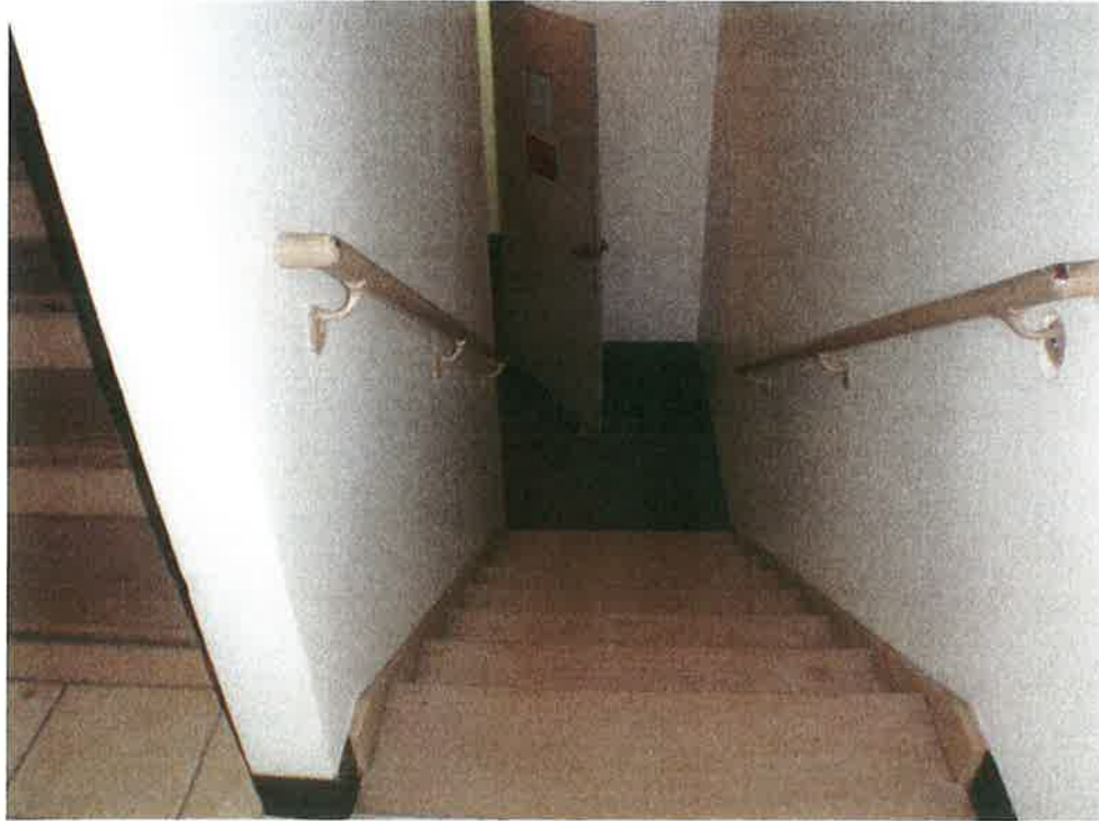
Heartland Building Wing A stairway
