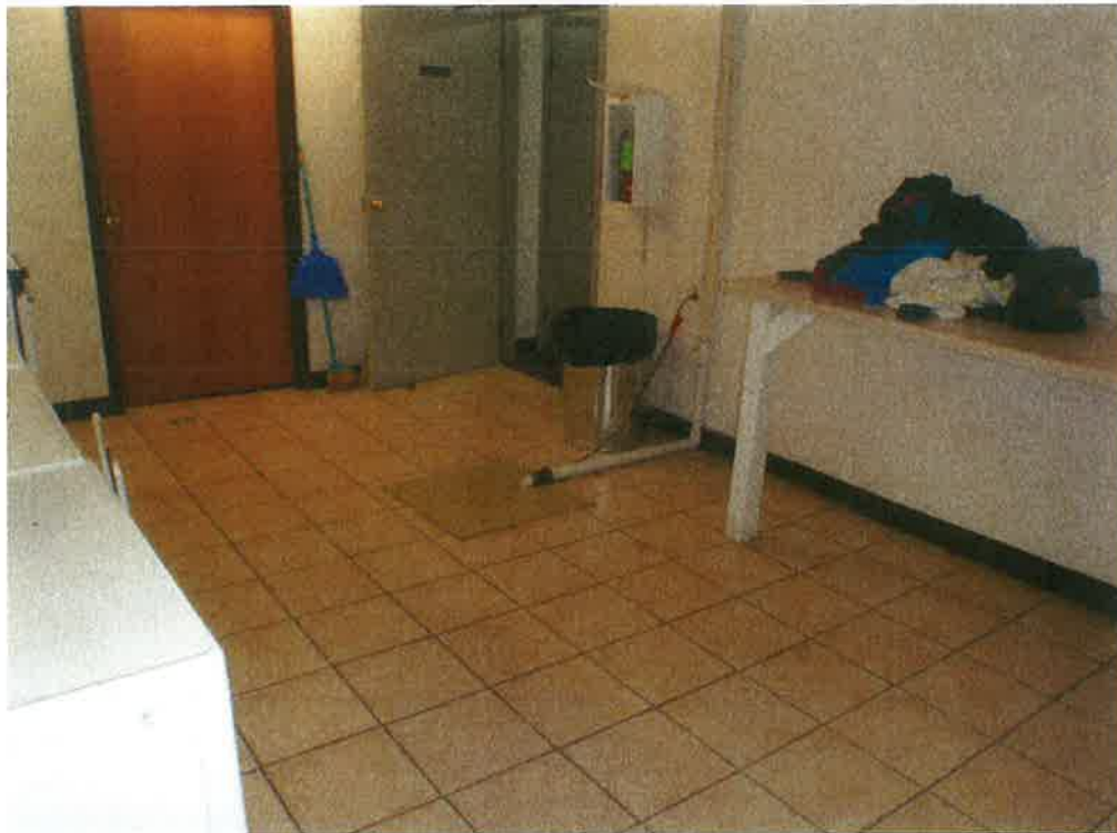
Heartland building – Wing A laundry room showing sump pump in floor
