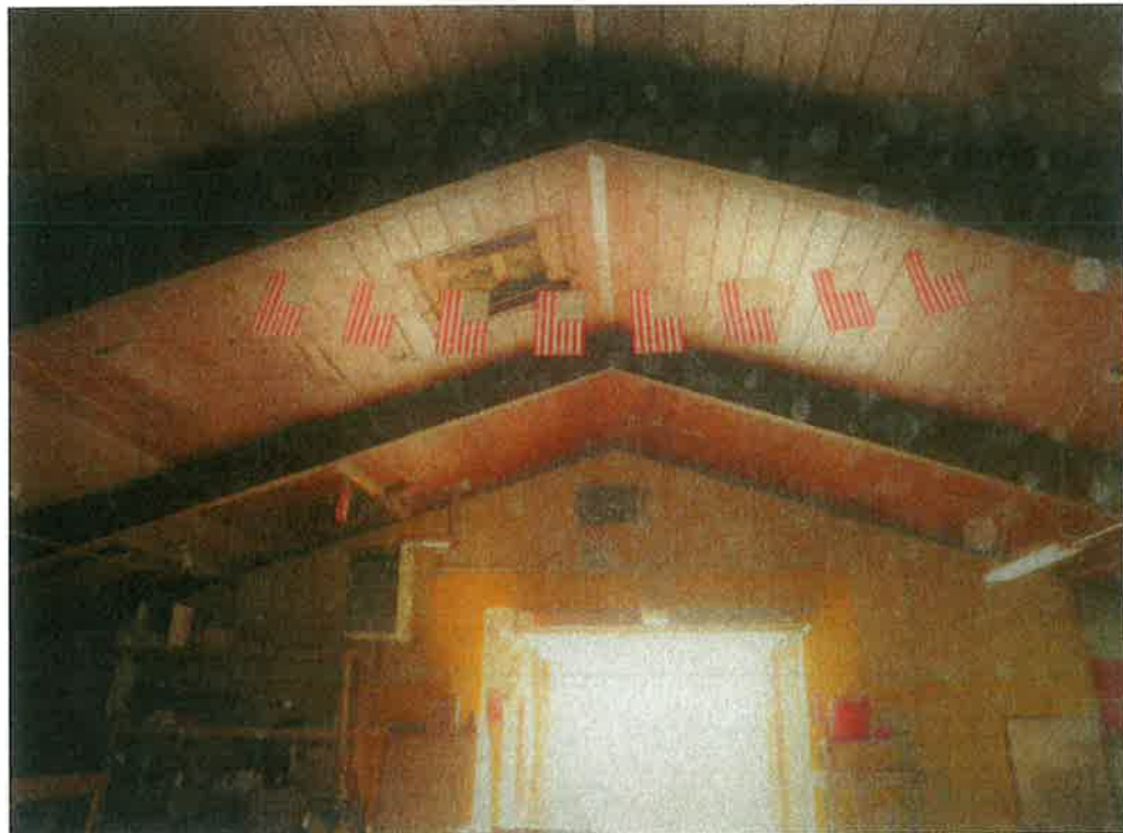
Former pool building – inside view
