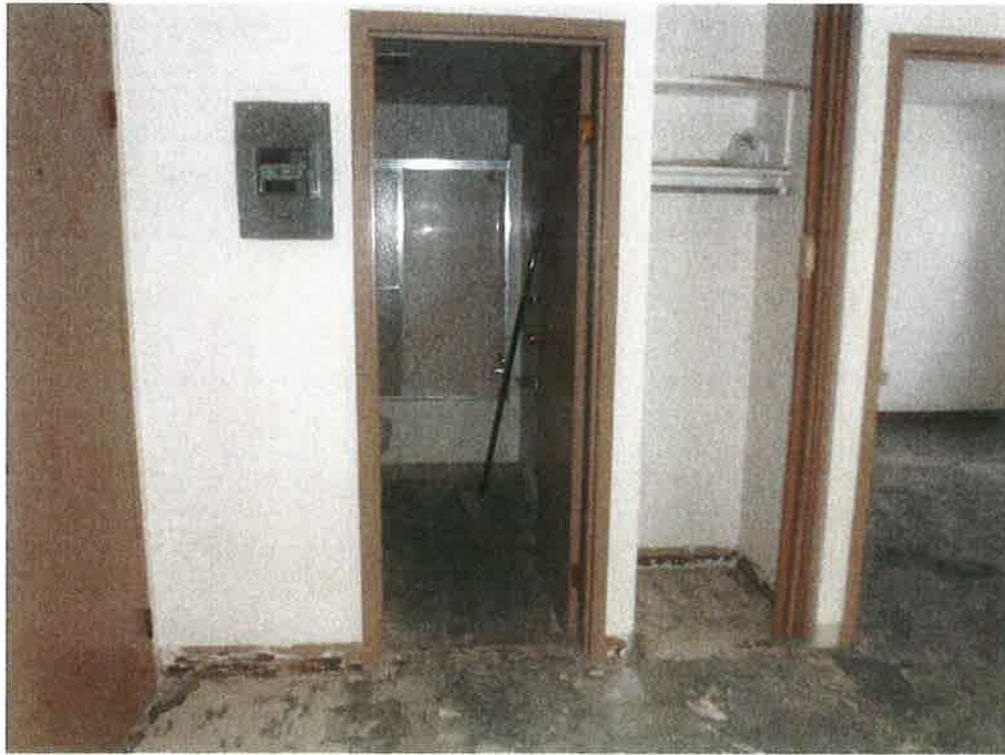
Heartland building – Apartment 4A with flooring removed by building owner
