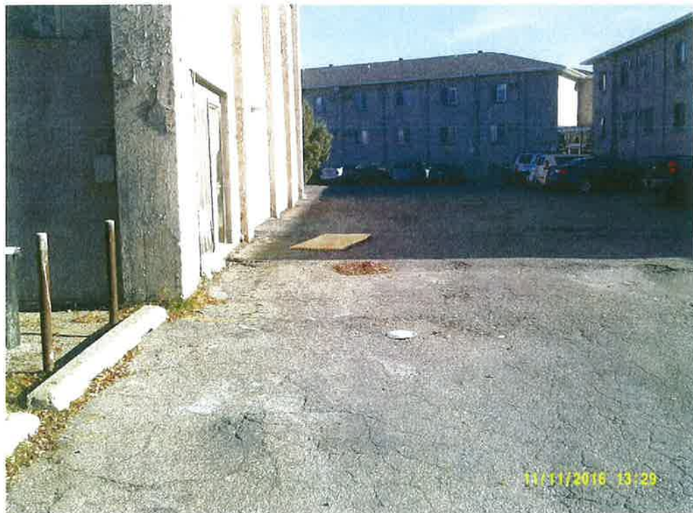
North storage building (left) – Heartland Building and north parking lot: asphalt heavily potholed, cracked and patched throughout
