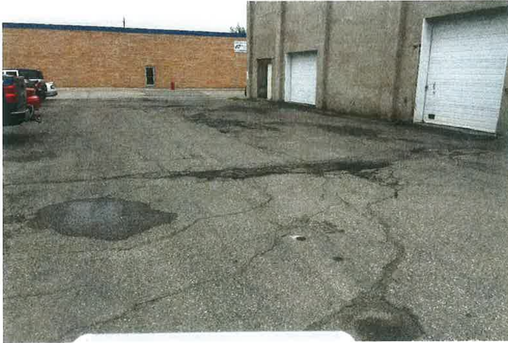
Heartland north parking lot - asphalt potholed, cracked and patched throughout
