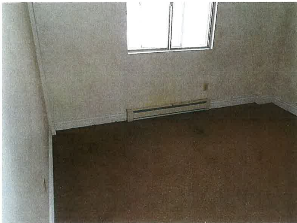
Heartland building – Apartment C12 – staining and cracks on exterior wall
