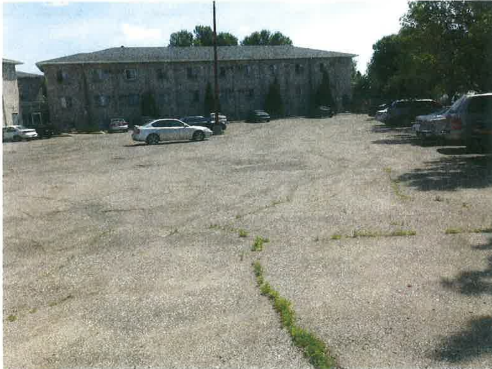
Heartland south parking lot view to the east – note numerous cracks in parking lot surface
