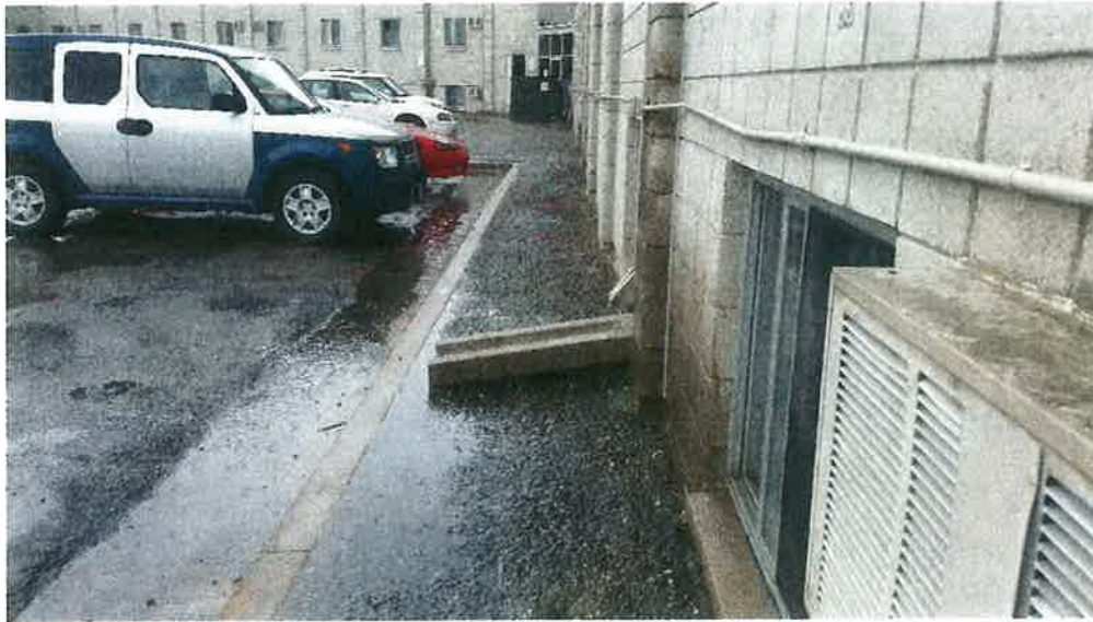
Heartland north parking lot showing drainage issues adjacent to building
