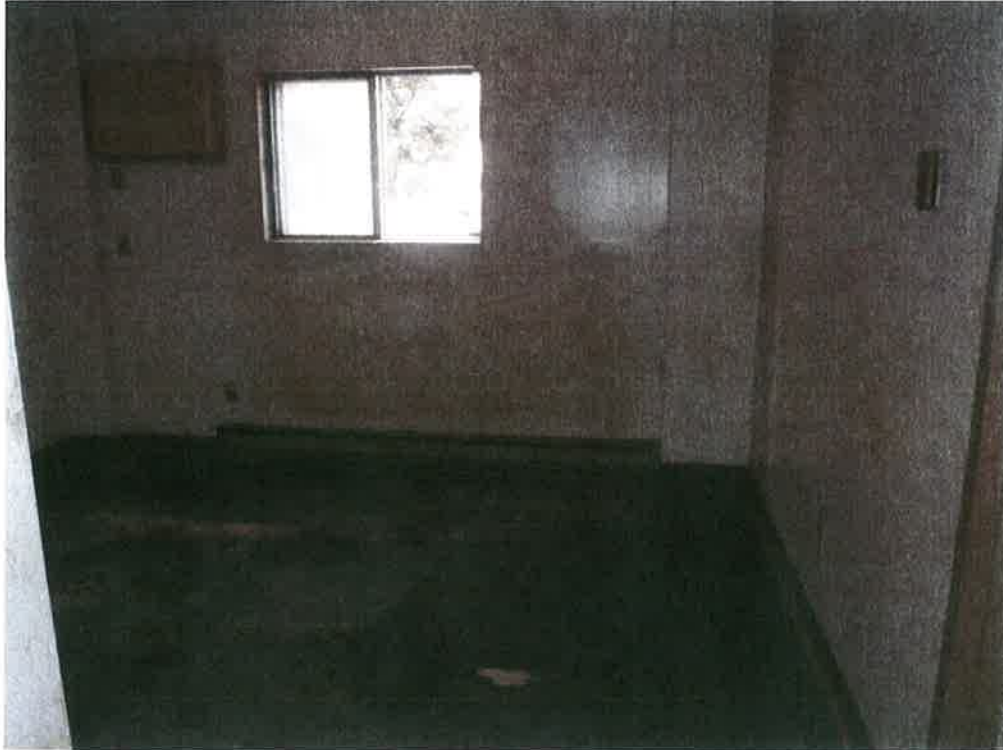
Heartland Building Apartment 10A – walls stained and condition is in overall poor condition
