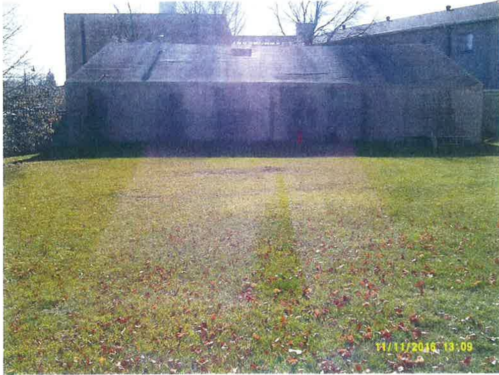
Heartland former pool building view to south – roofing/ceiling is starting to collapse and leaks
