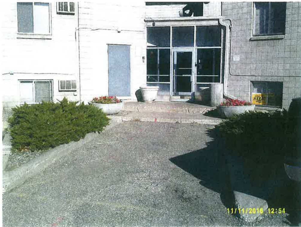
Heartland south parking lot building entrance – door latches and locks are in poor condition
