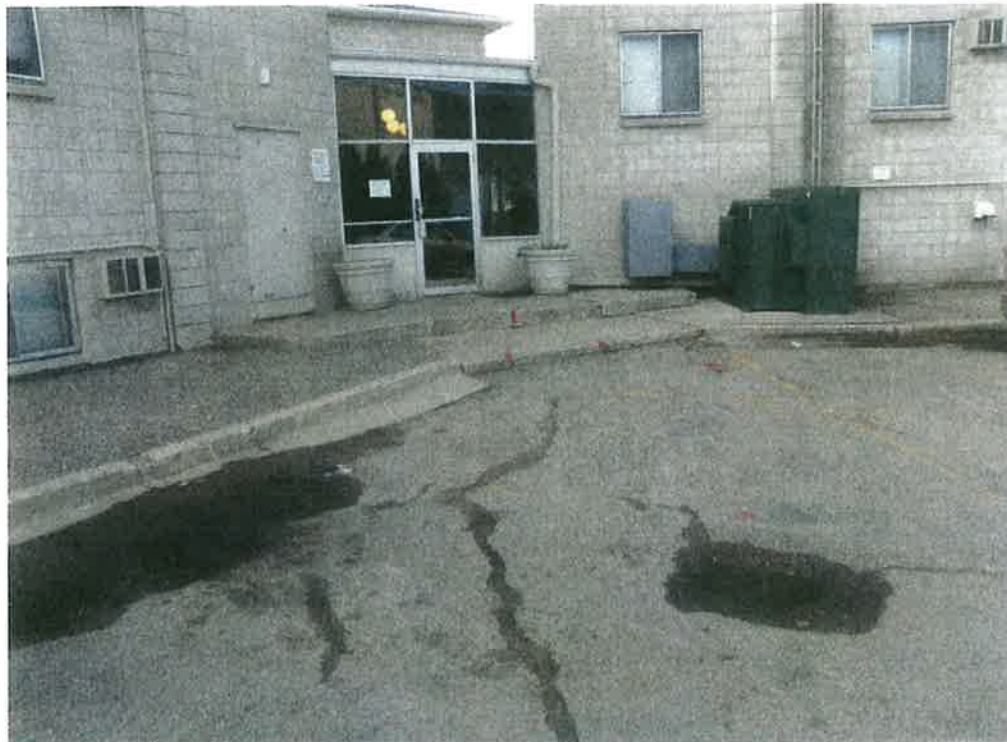
Heartland north parking building entrance - asphalt potholed, cracked and has settled throughout
