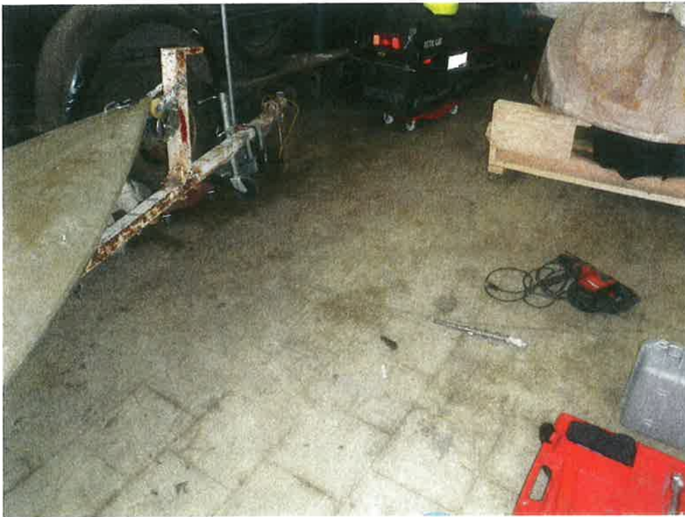
North storage building west side – asbestos floor tiles
