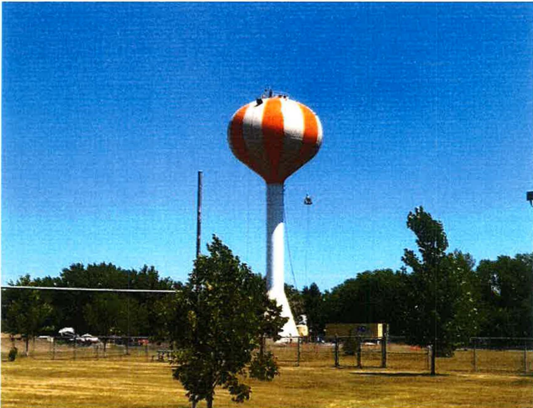
Painting crew from TMI Coatings, Inc. work on the exterior coatings on Water Tower #5. The picture was taken on July 14, 2017.
