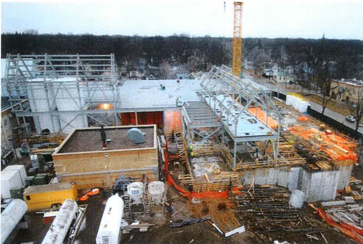
Site photo of the MWTP plant construction (March 2017). A primary reason for constructing the MWTP is Sheyenne River water quality. The reliability improvements under Project WA1510 will help transfer water from the Sheyenne River to the MWTP.
