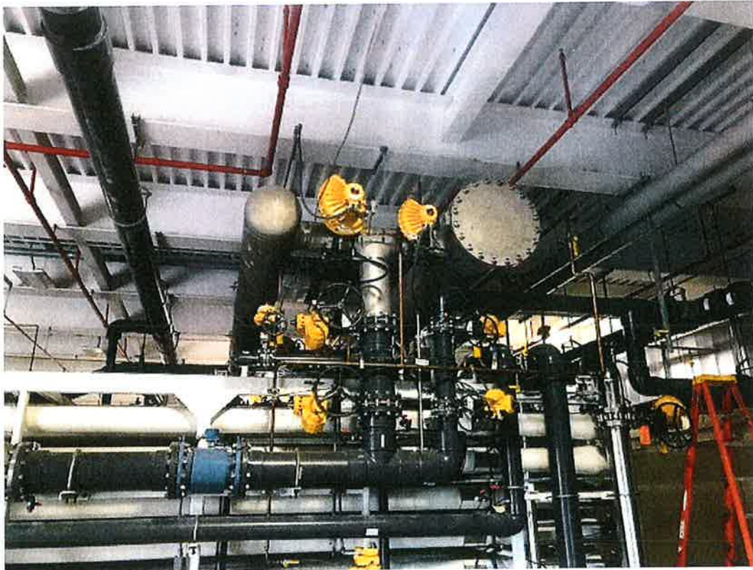
Piping, valves, pressure vessels, and other components on Reverse Osmosis (RO) skid. The RO system has two discharge headers (shown on top) to send RO water to the end of the MWTP or to softening trains in the existing water plant. Photo from June 2018.
